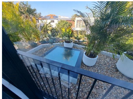
Figure 8: 9B unauthorised skylight.
