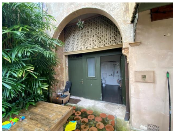
Figure 7: View of an existing bathroom within the partially enclosed driveway from the rear courtyard.
