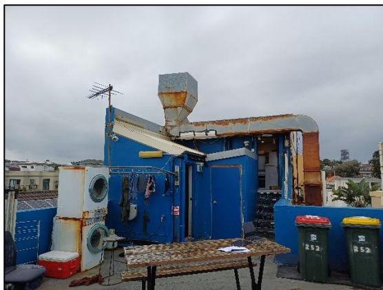
Figure 3: Existing structure on the roof
