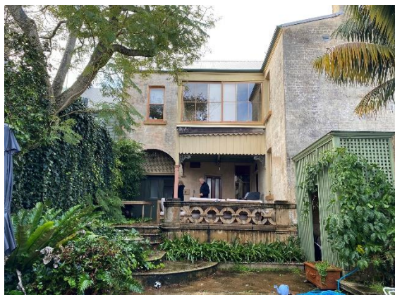
Figure 6: View of the terrace dwelling and landscaping from the rear courtyard.
