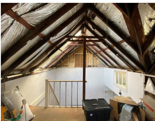
Figure 10: Existing mezzanine floor within the rear outbuilding.
