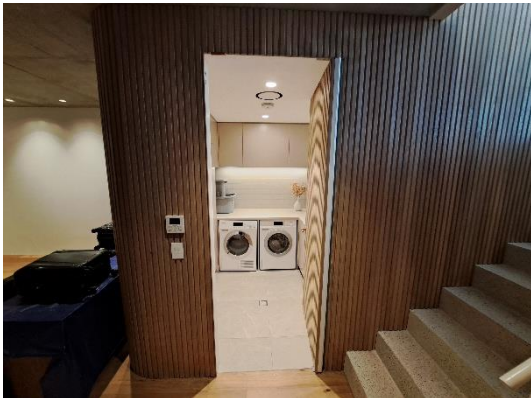
Figure 5: 9A unauthorised basement.
