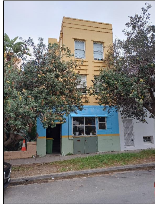
Figure 2: Subject site viewed from Ramsgate Avenue
