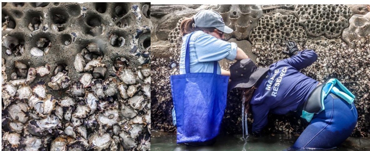
Figure 11. Ecological engineered habitat panels on a seawall. Photo by Aliah Banchik.
