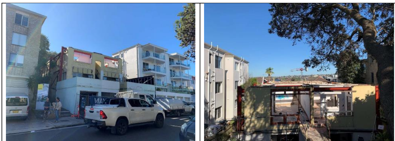
Figure 7 and 8: Site progress photo provided by the applicant showing the front and rear of the site. The roof and glazing have been removed and temporary support and cross bracing in situ.
