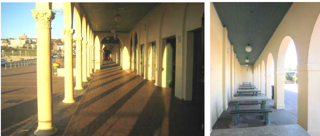
Figure 97 Views along the southern loggia (left) and western loggia with 1930s tables and benches (right). Early photographs show the floor of the southern loggia was originally concrete. The original margin beneath the columns has been retained. Loggias generally have retained timber soffit linings.
