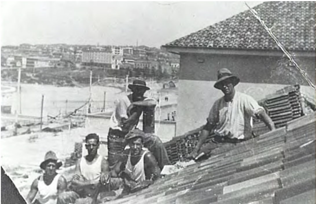
Figure 22 Men in the course of laying tiles on the roof of the Bondi Pavilion. The tiles are glazed in a variety of colours, evident in the range of tones across the sections of roof shown in the photograph, and have the semi-circular Cordova pattern that was popular during the interwar period. Source: WL Picnumb 586.
