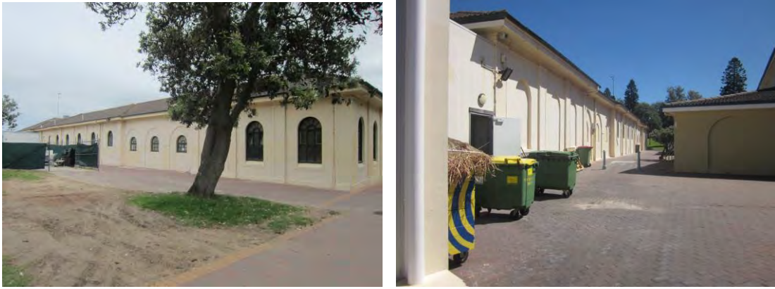
Figure 95 The western side of the Pavilion complex has been subjected to a relatively high level of change, including the enclosure of the pair of loggias and modifications to original window openings. Those on the beach side of the building have been blocked up or covered over).
