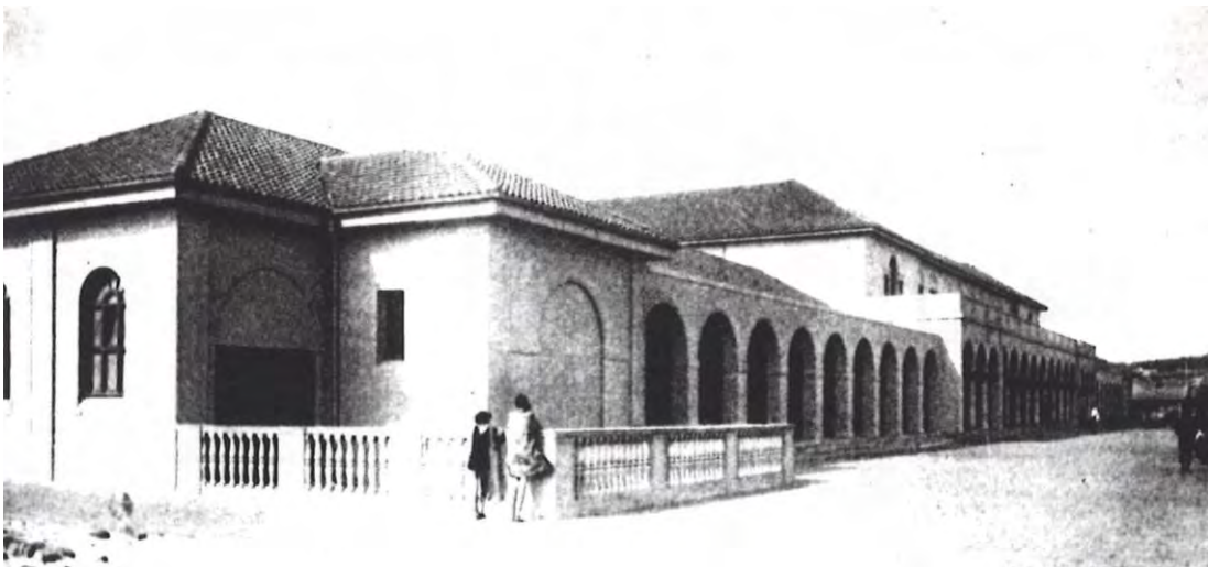
Figure 91 Circa 1930 photograph looking north along the principal facade of the Pavilion, showing the low balustrade that defined the entry to spaces then occupied by women's showers. The door opening has been modified and the blind arched panel formed into a door opening. Source: reproduced in The Home , April 1930.
