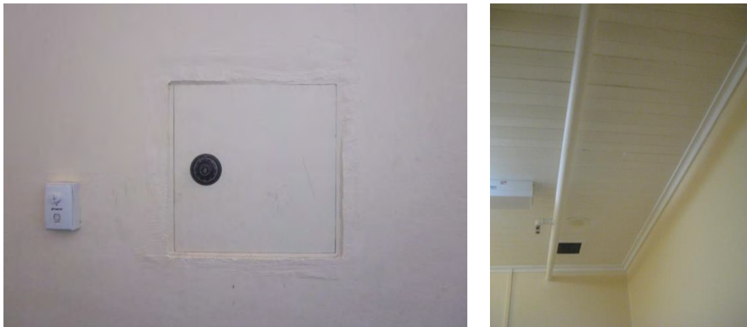
Figure 126 Intact early fabric in the eastern end of the first floor includes the safe mounted in one of the walls of the Ocean Room (left) and timber ceiling linings over the female lavatory (F7), located in spaces originally occupied by a lavatory and a storeroom. There are also early ceramic wall tiles in part of the female lavatory.
