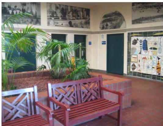
Figure 112 The former bathing costume/towel hire area and light well have been modified and opened up on its eastern side to become an atrium. The well-intentioned brick planter is an inappropriate element within the space. Interpretive photographs have been mounted around the space. Quarry tiles covering the floor are not original.
