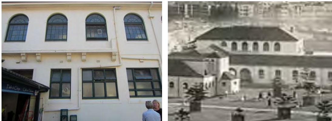
Figure 105 Evidence of a removed balconette on the north-eastern elevation. The absence of a sill moulding at the base of the three windows above the remnant balconette suggests that these may once have been door openings. The archival photograph (right) indicates the presence of the balconette during the 1930s.
