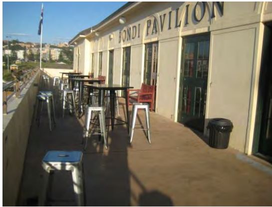
Figure 98 First floor terrace overlooking Bondi Beach and its environs. Its floor is covered with a trafficable waterproof membrane (left); concrete roof tiles are not original. Differing tones of individual tiles suggests replacement due to damage (right).
