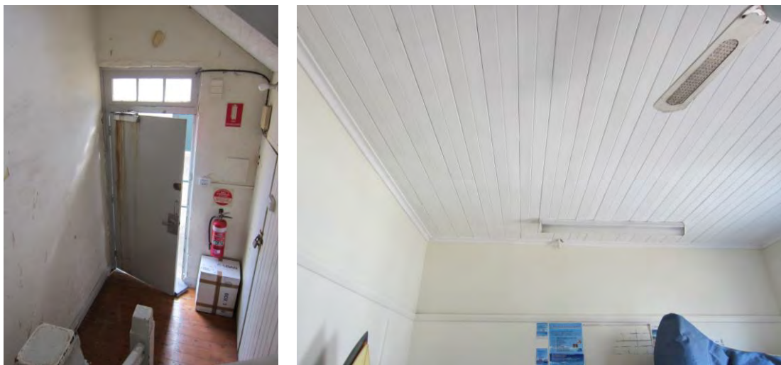
Figure 132 Ground floor vestibule associated with the stair to the former caretaker's flat (left, G45). The first floor spaces largely have timber board lined ceilings (right), although some have battened sheet linings, possibly of fibrous plaster.
