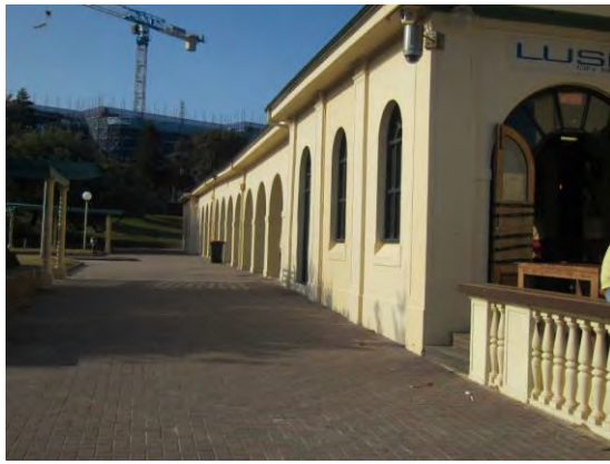
Figure 92 Looking north along the south-western facade. The balustrade has been modified to provide access to the tenancy space that now occupies the shower room (left). The south-western facade incorporates a secluded loggia (right).
