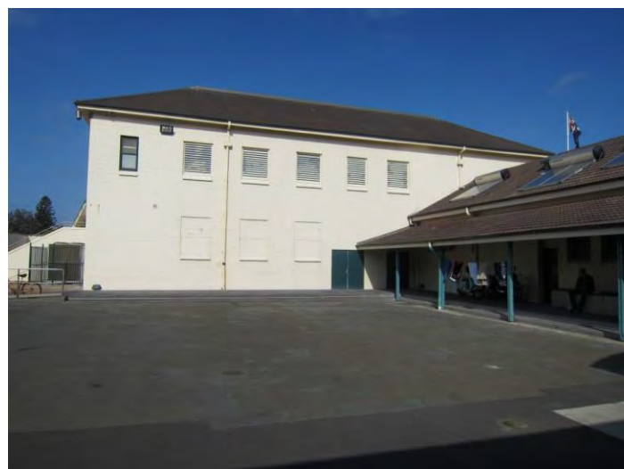
Figure 100 Western end of the Main Pavilion. The external fabric of this section of the building was replaced, probably when the theatre was installed during the 1970s. This resulted in the loss of important original detail and fabric. Compare to Figure 101.
