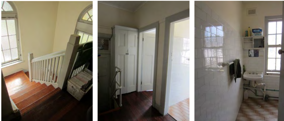
Figure 133 The first floor of the Auditorium pavilion has retained a substantial amount of original fabric including its stair (left; F28), doors, a cupboard, skirting boards and picture rails (centre; F27). However, the bathroom has been refurbished (right; F24).
