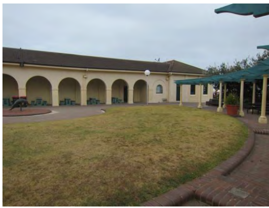
Figure 92 Looking north along the south-western facade. The balustrade has been modified to provide access to the tenancy space that now occupies the shower room (left). The south-western facade incorporates a secluded loggia (right).
