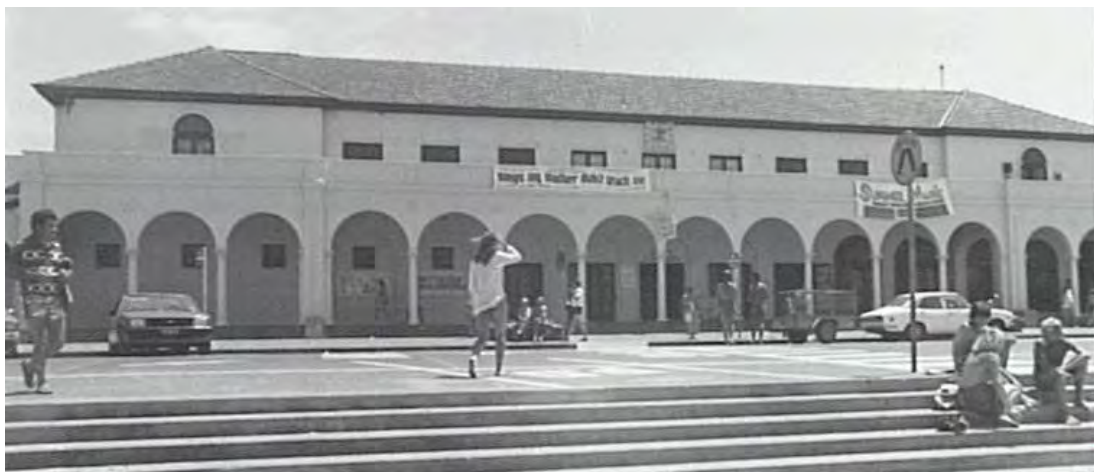
Figure 88 This 1980 photograph shows the configuration of original fenestration associated with the Turkish Bath on the western side of the principal facade and the door openings associated with retail tenancies on its eastern side. The recent arched openings in the western section of the elevation have been undertaken in a sympathetic manner, echoing the openings associated with the eastern retail spaces that already existed.
