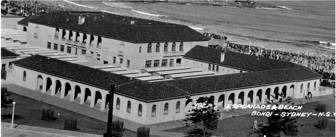
Figure 101 Part of a 1930s postcard, which clearly shows the original appearance of the western section of the Main Pavilion and the absence of a verandah attached to the single storey wing that housed the Turkish Bath. The verandah was subsequently constructed towards the end of the 1970s.
