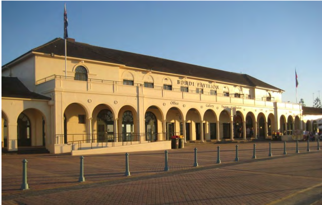
Figure 87 Principal elevation of the Bondi Pavilion in March 2015. Modifications include ramps, arched openings in the western section of the elevation, addition of signage above first floor windows, ramps and the handrail above the balcony balustrade wall coping. Signage mounted on wall surfaces is also relatively recent.
