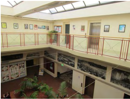
Figure 122 Upper level of the Atrium (F10), originally a light court and modified by the construction of a perimeter mezzanine and enclosed by translucent vaults.
