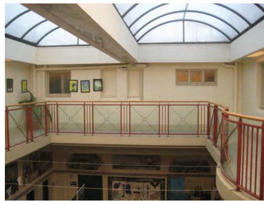
Figure 122 Upper level of the Atrium (F10), originally a light court and modified by the construction of a perimeter mezzanine and enclosed by translucent vaults.
