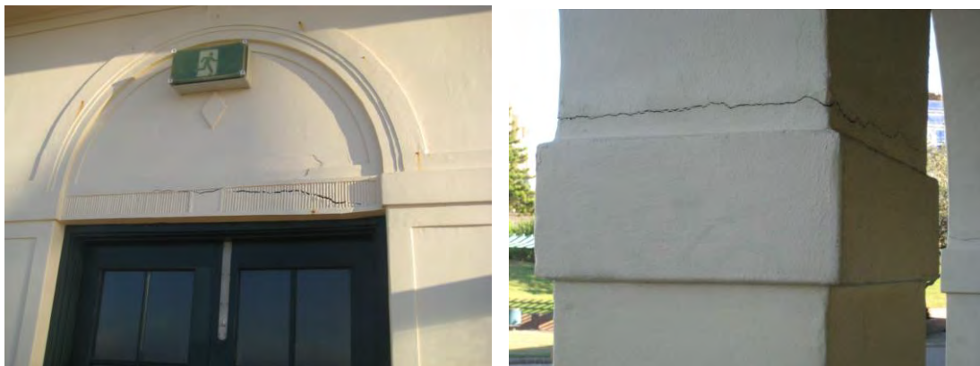
Figure 106 Cracking in rendered wall surface above a first floor door opening on the southern side of the Pavilion (left) and in a pier associated with the loggia on the south-western side of the building (right) is indicative of movement in the building structure, which is common to many buildings.
