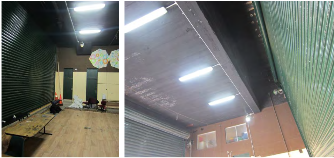
Figure 131 Stage area within the early 1930s Stage Pavilion. The former caretaker's residence above, now used for office purposes, only extends over part of this space and has a reinforced concrete floor slab supported off a deep reinforced concrete beam.
