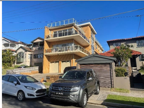
Figure 3: Neighbouring residential flat building to the south of the subject site (No. 302)
