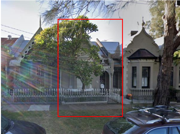
Figure 1: Subject site (in red) viewed from St James Road.
