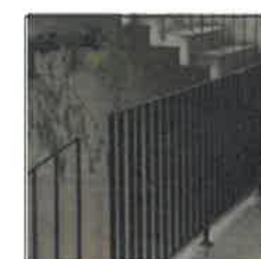
9. BAL POWDERCOAT ALUMINIUM BALUSTRADE INTERPON "SABLE BASS"
