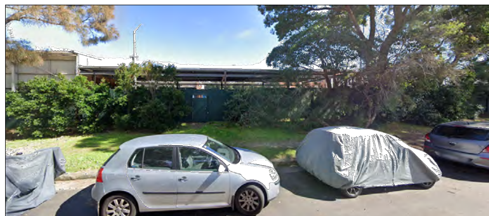
Bus Depot Side façade
