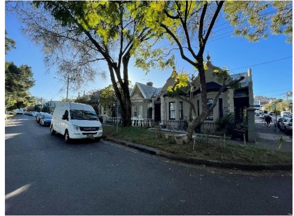
Figure 2: Street context of St James Road, looking north.
