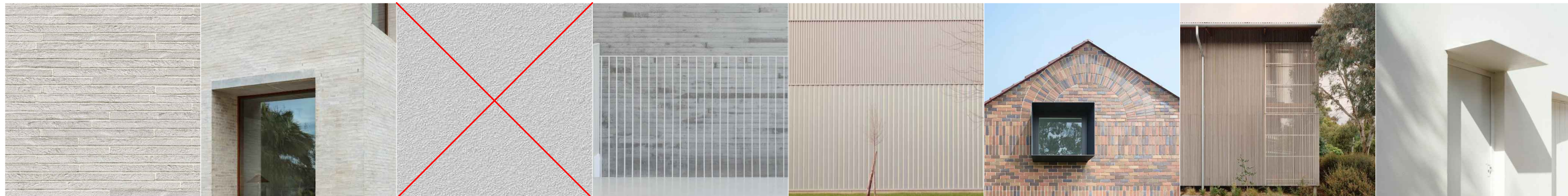
A White Brick B Brick Sills C White Render D Steel Balustrade E Corrugated Steel Clad F Steel Window Shades G Timber Screen H Steel Hood
