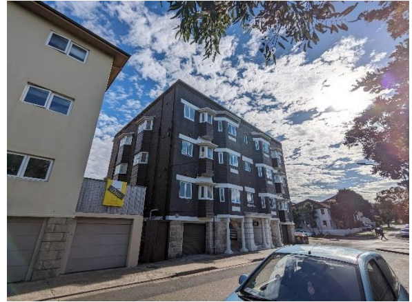
Figure 2: Site viewed from Gould Street, looking north.
