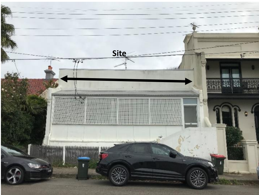
Figure 2: View of 19 Prospect Street and adjoining developments, looking west
