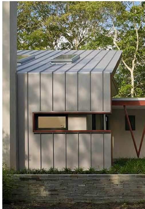
1 Roofs & side taped walls sample
