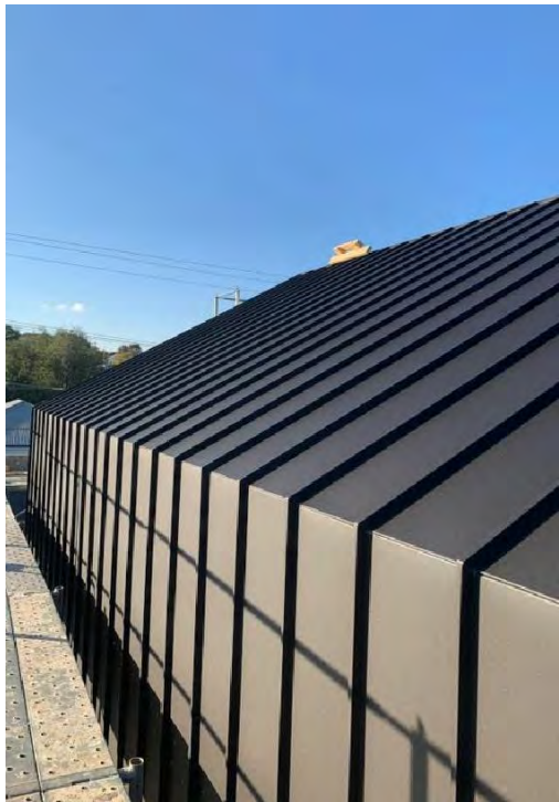
1 Roofs & side taped walls sample
