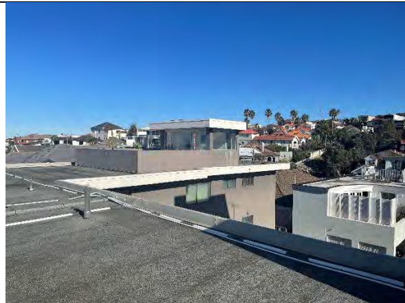
Figure 3: Existing terrace located on the roof
