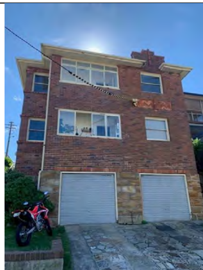
Figure 2: Neighbouring RFB to the west at No. 132 Hewlett Street, facing north
