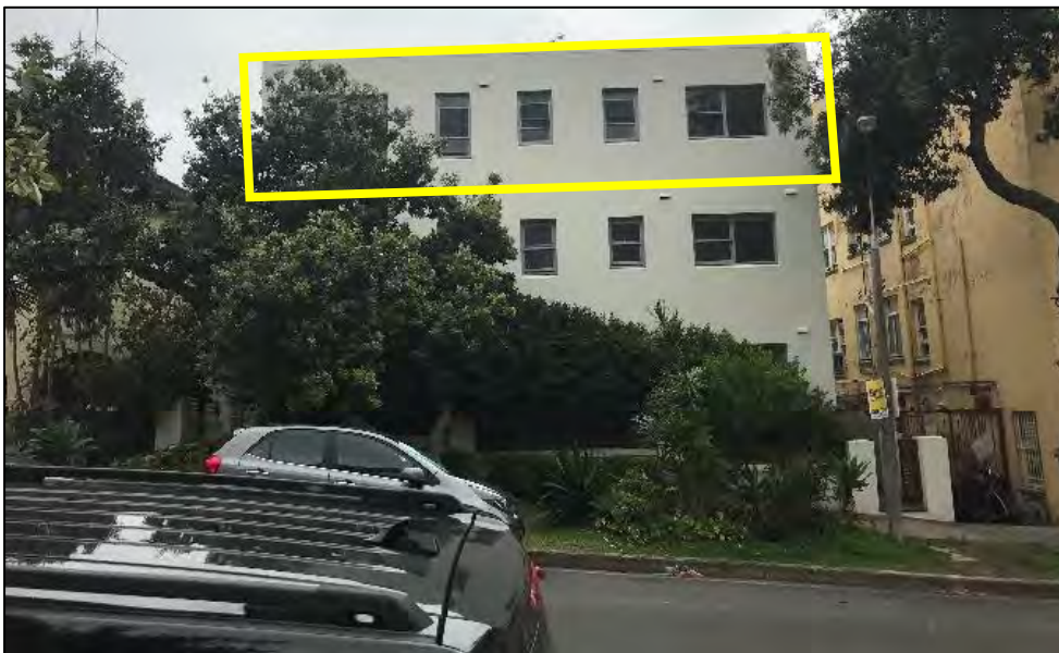
Figure 2: Front of the subject building (unit 15 outlined yellow) as viewed from Francis Street, looking north-east.
