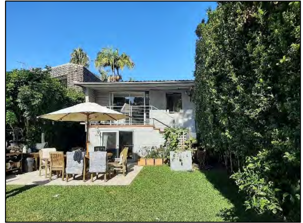
Figure 2: Rear elevation of the dwelling
