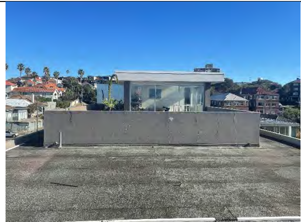
Figure 4: Existing terrace located on the roof
