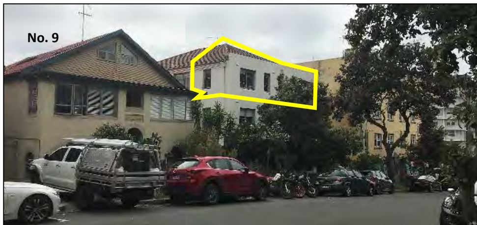
Figure 3: Front of the subject building (unit 15 outlined yellow) as viewed from Francis Street, looking east.
