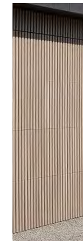
VERTICAL BATTEN - ALUMINIUM (NON-COMBUSTIBLE) GARAGE DOOR
