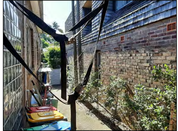
Figure 9: Existing eastern side boundary setback looking toward the rear of the site (north) showing windows on the subject site (left) and opposing windows on the side elevation of 398 Bronte Road
