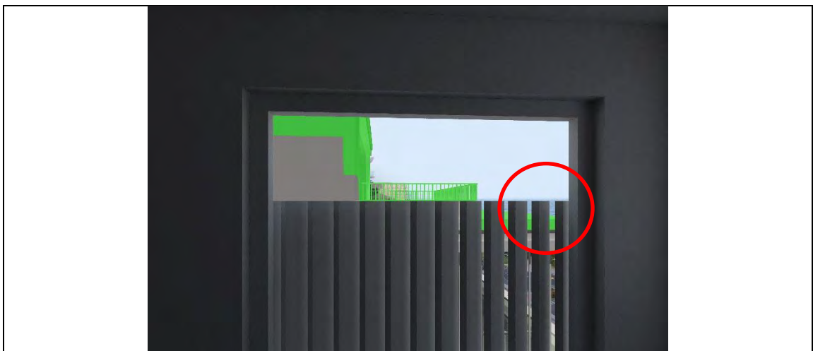
Figure 13: Views from the approved east facing dormer (viewpoint 01), height variation shown in green Source: Urbaine Design Group
