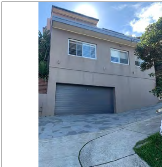
Figure 1: Subject site frontage, facing north
