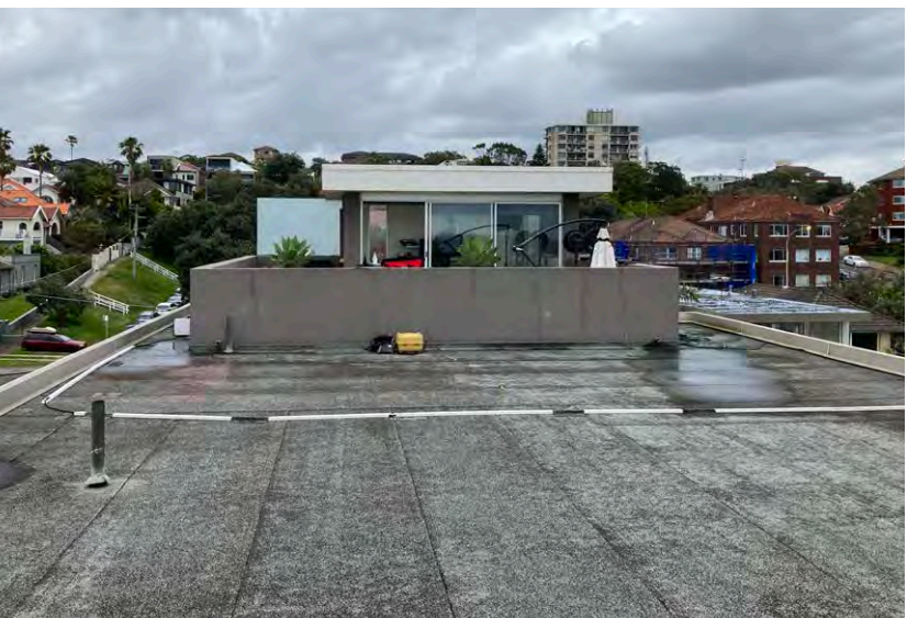
VIEW D FROM ROOF LOOKING WEST TO ROOF PAVILION
