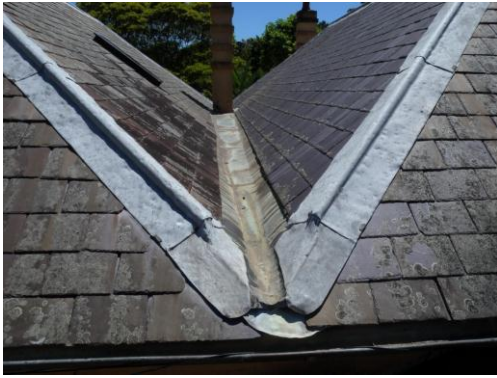
Figure 2. 85: Main Wing tapered gutter
