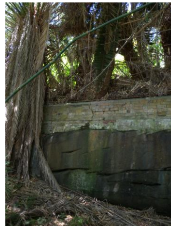
Figure 2. 115: Later addition brick wall to rocky outcrop (SF43A)
