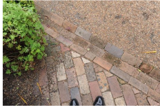
Figure 2. 109: Detail of brick guttering to drive (SF10)
