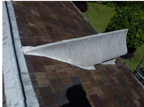
Figure 2. 82: Ogee vent over Kitchen
