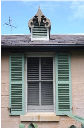
Figure 2. 71: West elevation window (W21) with ogee vent above
