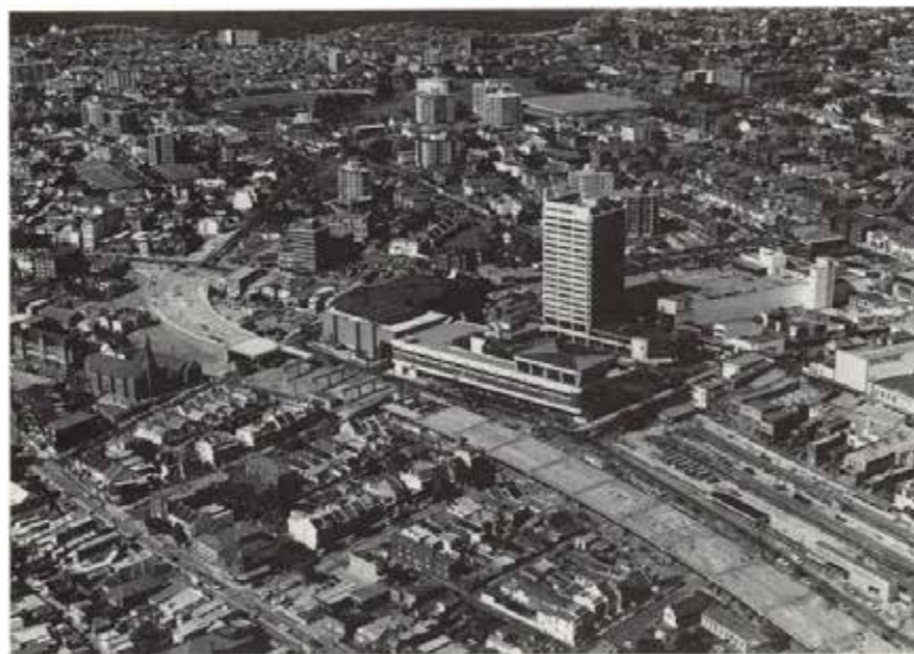
The viaduct is nearing completion in late 1978
