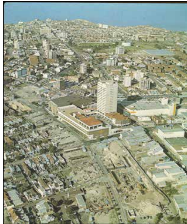
Aerial view of early construction work on the Bondi Junction bypass in 1977
