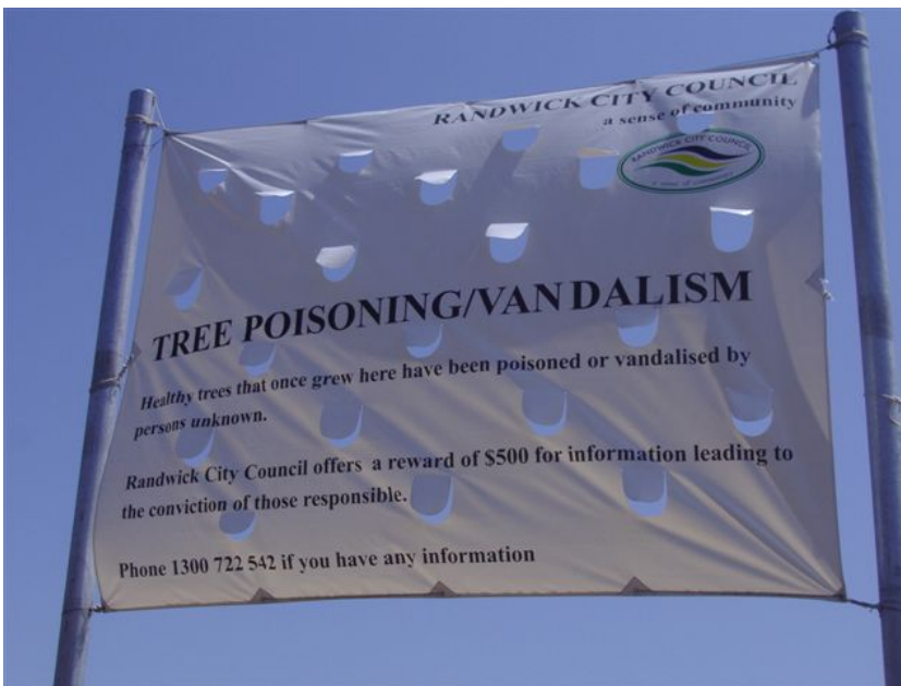
Shroud and banner erected at Grant Reserve Coogee by Randwick Council (Note the air vents to reduce wind impact. The structure is 6 metres in height and the shroud is attached with stainless steel buckles and wire to 100mm galvanised steel posts.)
