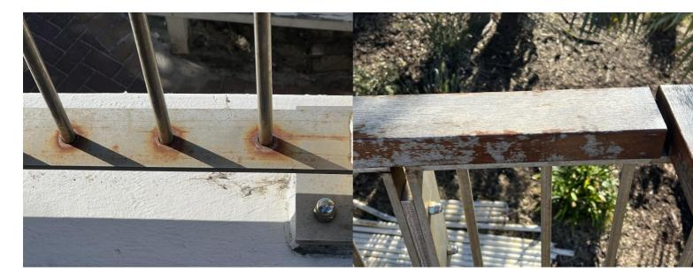
Putting any flat steel at an angle would also help. Note round steel bars are less expensive than the current design.
