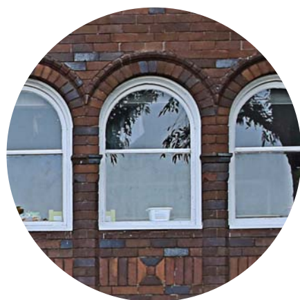
> Brick arch with brick label course
