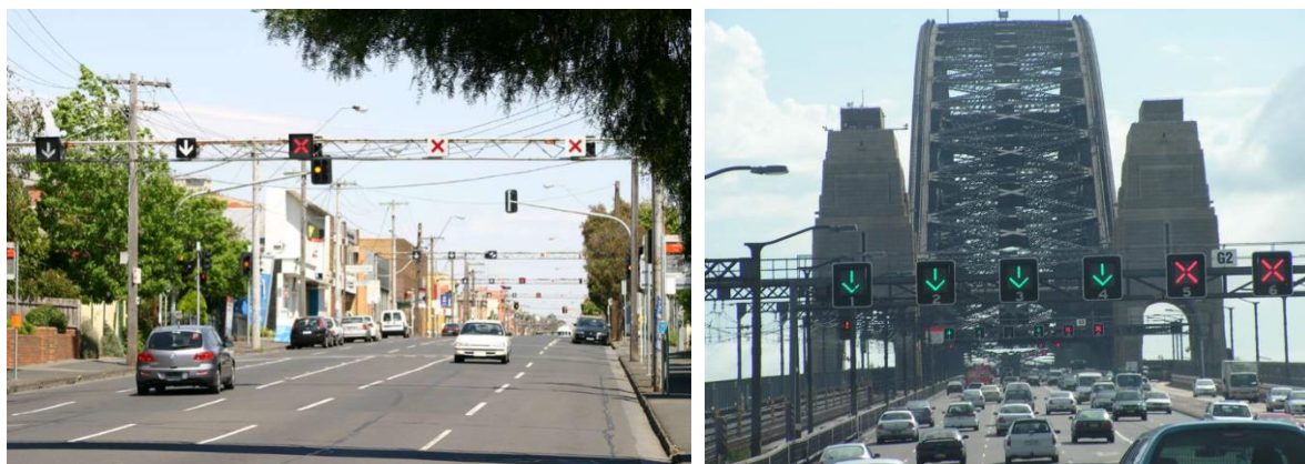
Photo 8.1 Lane management using overhead lane indicators
