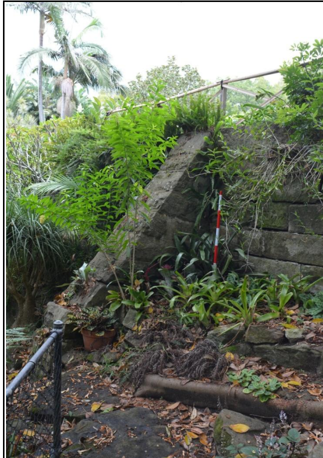
Figure 5.7: Most if not all of this sandstone will have been cut and shaped on-site. The form of the original platforms at the head of the gully and its shelving sides with no doubt some rock overhangs of different sizes at different levels are now hard to imagine
