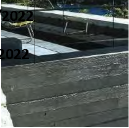
5. SALVAGED EXISTING SANDSTONE 6. HORIZONTAL BOARD FORMED CONCRETE WITH GLASS BALUSTRADE
