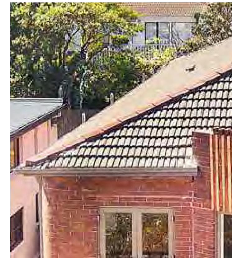
TL:01 ROOF TILE TO MATCH EXISTING
