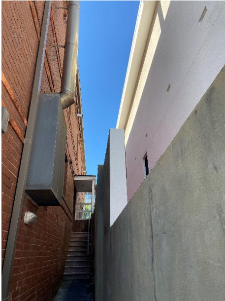
Figure 6: View of stairs to entry of building and southern side boundary fence, looking east along southern side setback
