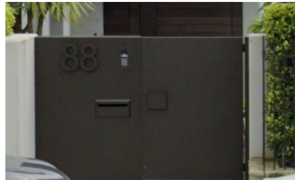
MF - METAL PRIVACY FENCE ON WITH WHITE CEMENT RENDERED WALLS ADJACENT. COLOUR TO MATCH CR2.
