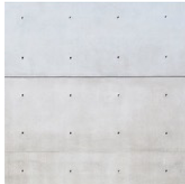
2 OFF-FORM CONCRETE - OFC
