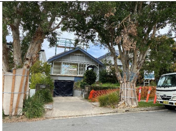
Figure 3: No. 30 Yanko Street currently under construction, facing south
