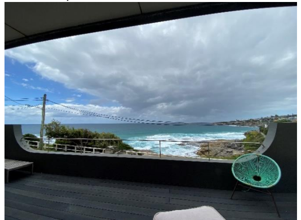
Figure 4: Existing front balcony/ deck area on the first level
