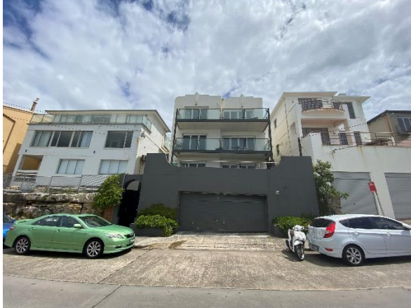
Figure 1: View of site and adjoining properties looking north from Gaerloch Avenue
