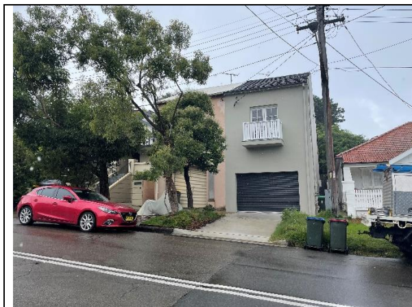
Figure 2: Subject site viewed from St Thomas Street
