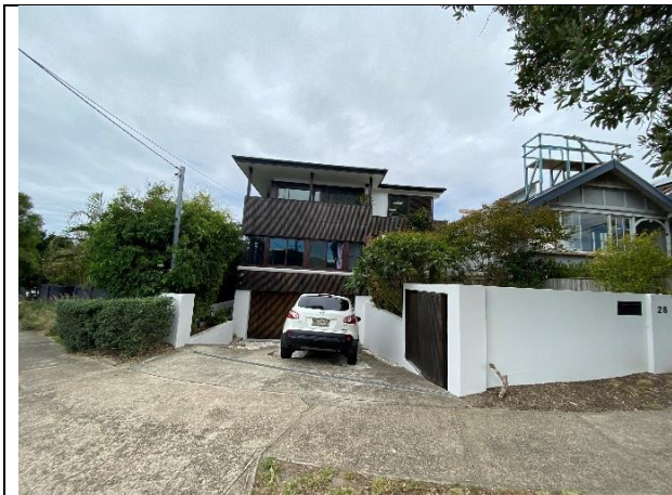
Figure 1: Subject site frontage facing south, neighbouring dwelling under construction west
