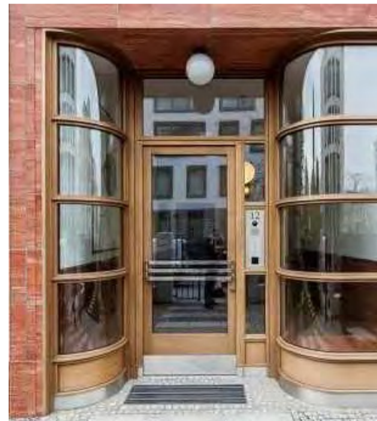
TM:02 GLAZED TIMBER FRAME WINDOW AND DOORS
