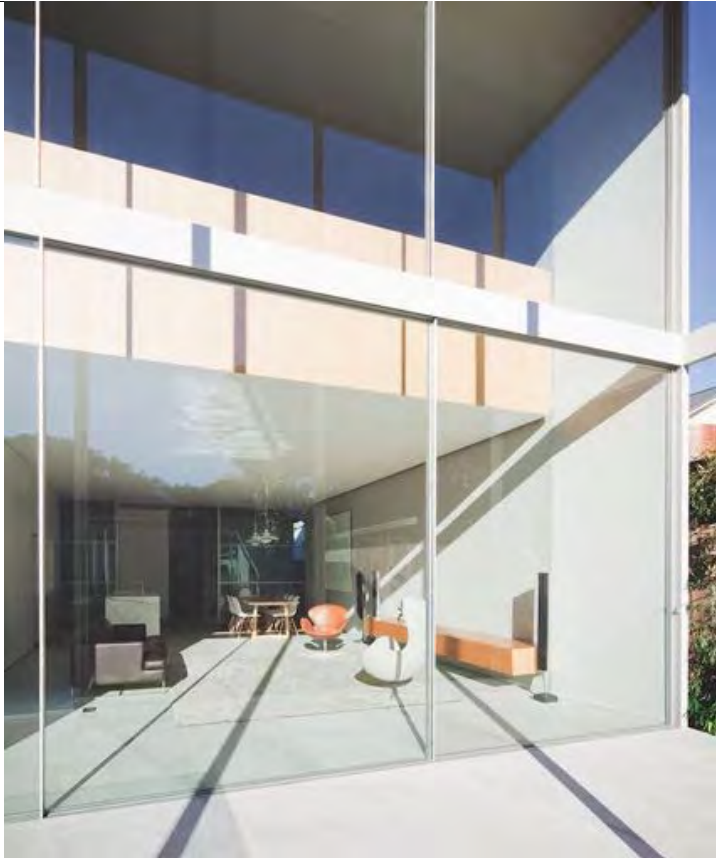
Aluminium framed clear and frosted, fixed and openable glazing - White colour
