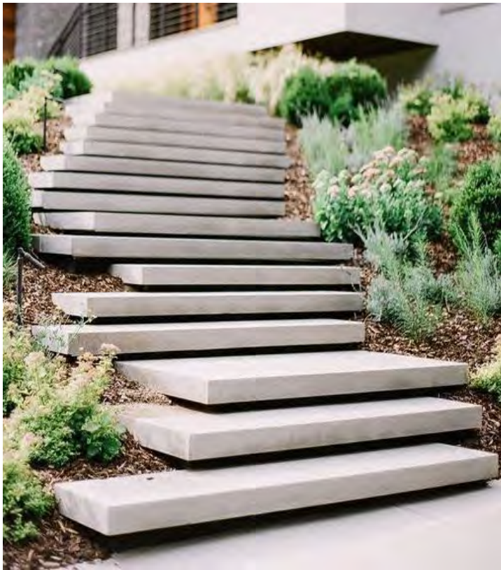
Off form finish concrete steps and seats - Standard concrete colour
