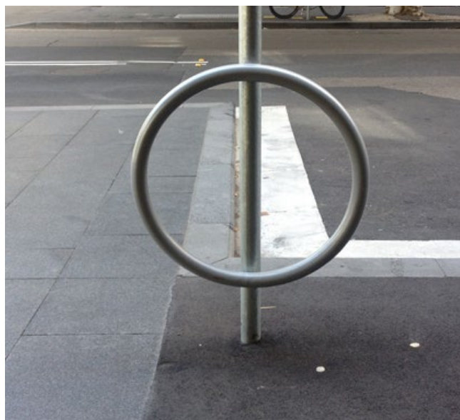
Bicycle Hoop attached to street signage pole
