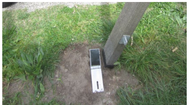
Recycled Plastic Bollard Type B - Removable, showing removable socket and locking mechanism
