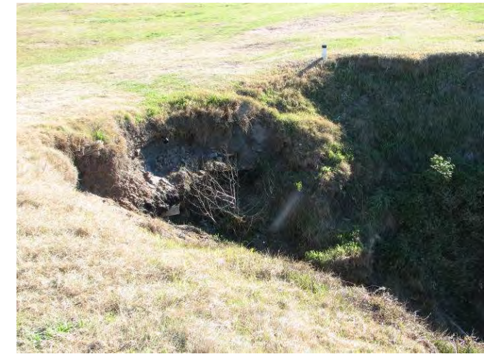
Instability of soil slope
