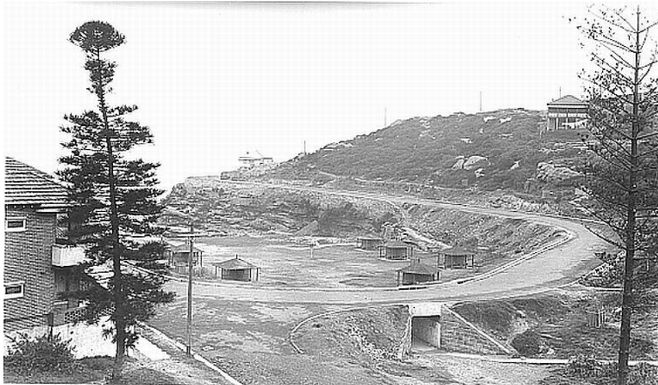
Figure 2.21 Tamarama, 1935. During the Great Depression road workers were employed under a government publicwork scheme to construct Marine Drive. The tunnel which once linked Tamarama Park with Tamarama Gully can be seen. (Source: Waverley Library Fact Sheet)
