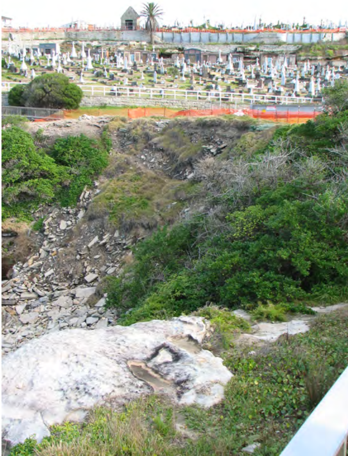
Figure 5.7 Fill batter slope at Waverley Cemetery
