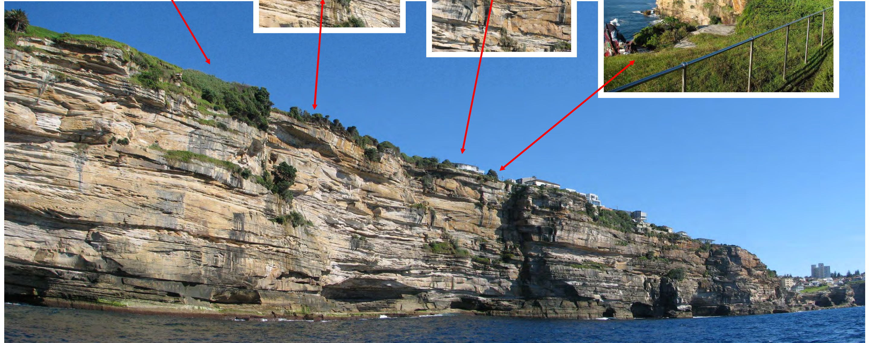
Cliff face below Hunter Street, Lancaster & Myuna Road
