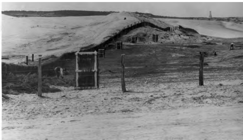
Figure 2.5 View north showing brush fences and tree planting 1900 (Source: Waverley Council)
