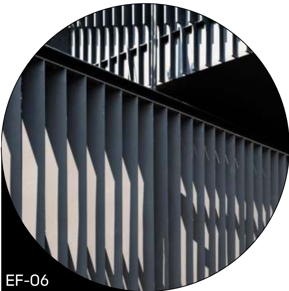
palisade battened screen for services
