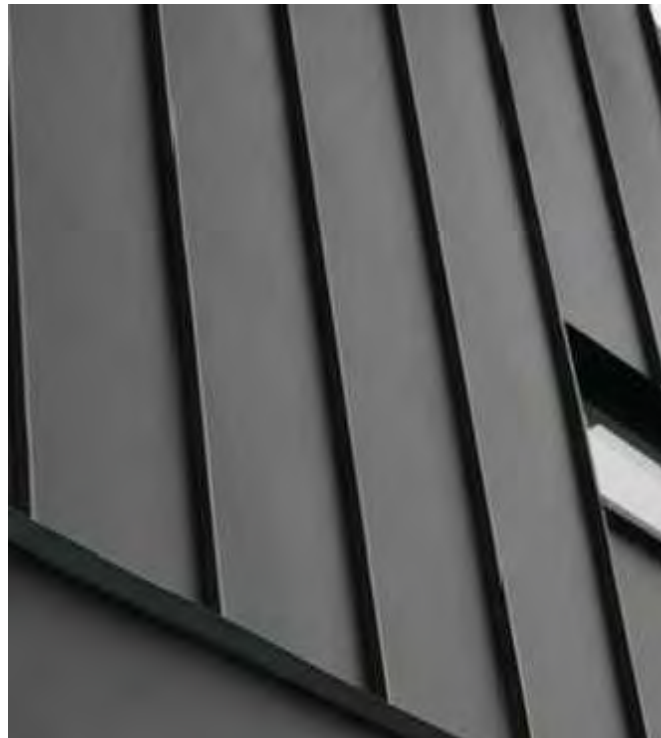
1 COLORBOND ULTRA METAL CLADDING / ROOFING
