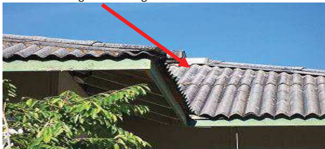
Asbestos corrugated roofing
