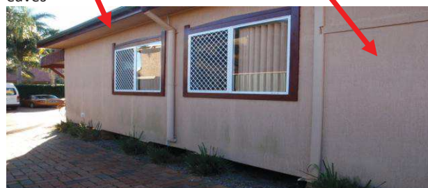
Asbestos cement sheet (fibro) used as lining for walls and eaves
