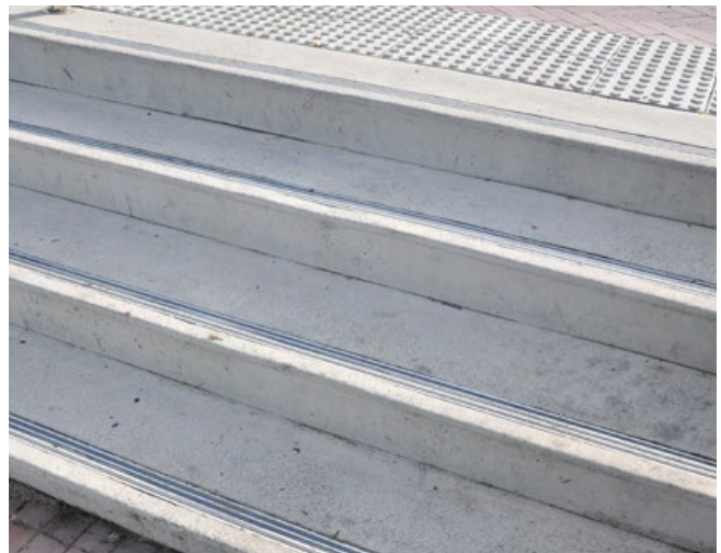
Stair Type A - Concrete
