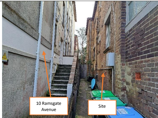
Figure 3: Side passage view of the subject site adjacent to 10 Ramsgate Avenue
