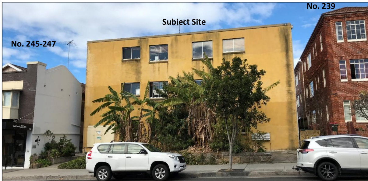
Figure 2: Subject site viewed from Bondi Road, looking south.
