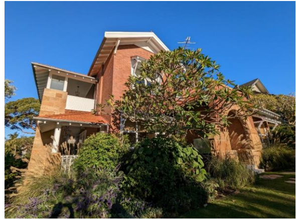
Figure 2: Existing dwelling viewed from within front setback, looking east
