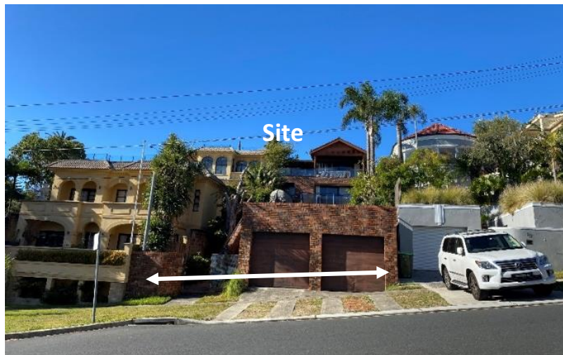
Figure 1: View of site and adjoining developments, looking east on Gilbert Street
