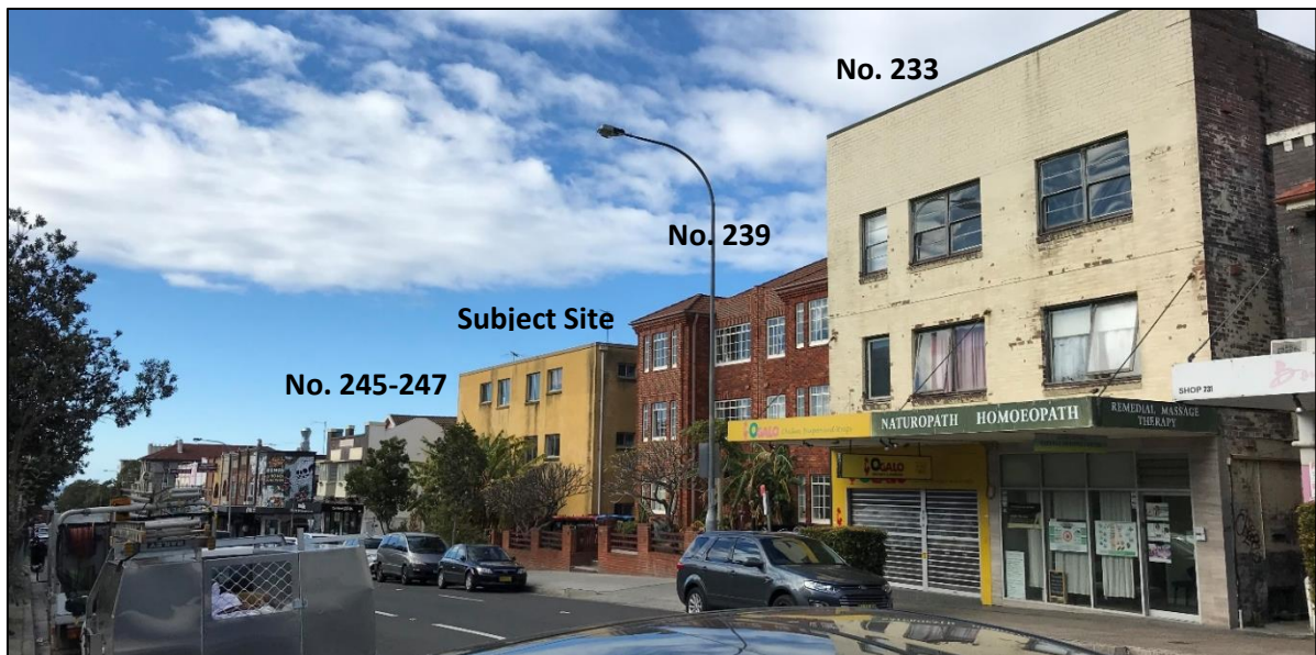
Figure 1: Subject site in context with Bondi Road, looking east.
