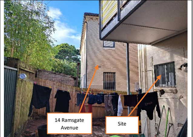
Figure 6: Rear view of the subject site looking towards 14 Ramsgate Avenue.
