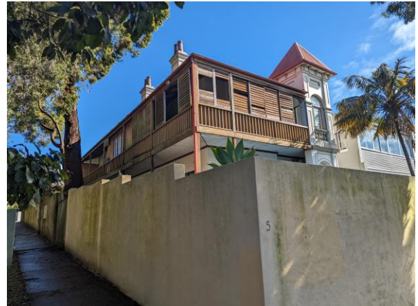
Figure 2: Site viewed from corner of Flood Street and Bon Accord Avenue, looking north-west
