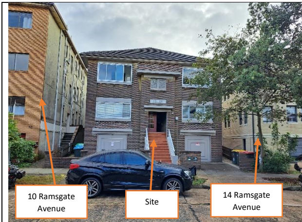
Figure 1: Streetview of the subject site
