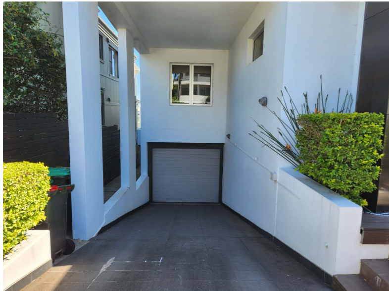
EXISTING SITE PHOTOS:
