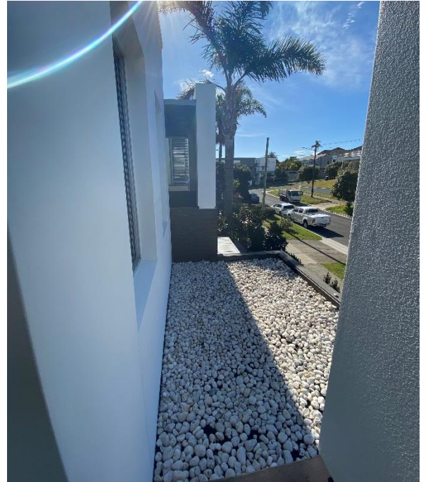
Figure 4: Photo taken from the southern first floor balcony facing north.
