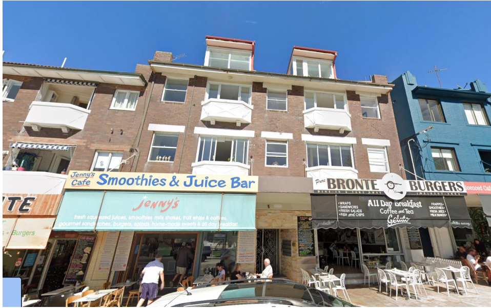
Figure 1: Site viewed from Bronte Road looking south-west. Image from Google Streetview
