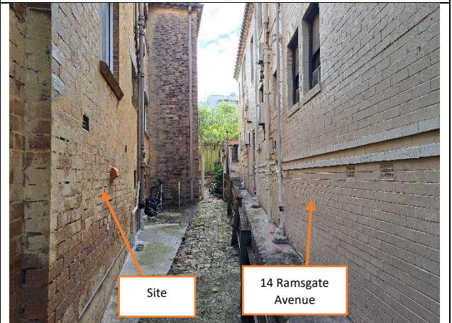
Figure 4: Side passage view of the subject site adjacent to 14 Ramsgate Avenue
