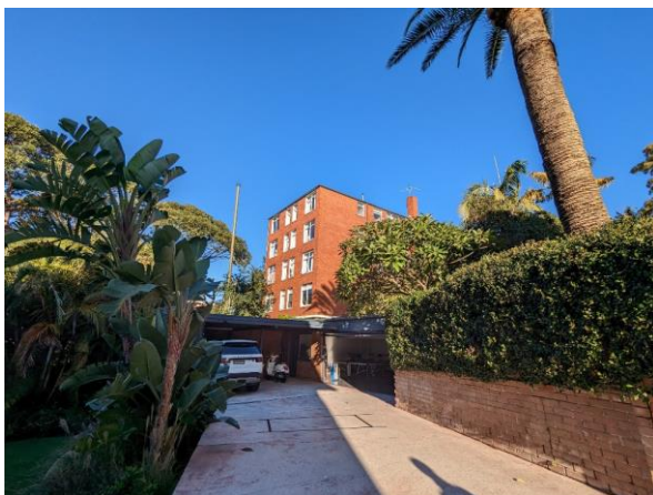
Figure 5: Existing carport and garage viewed from rear driveway, looking east
