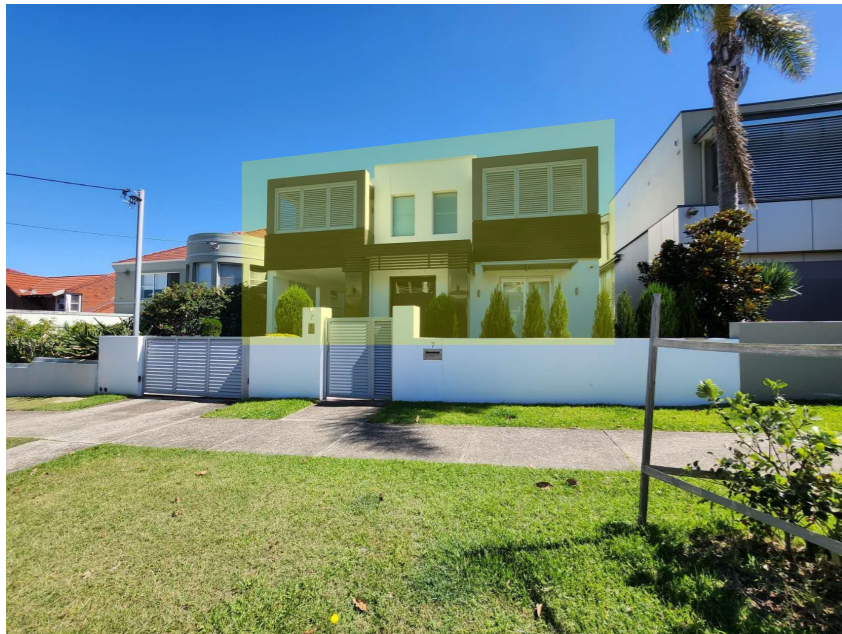
EXISTING SITE PHOTOS:
