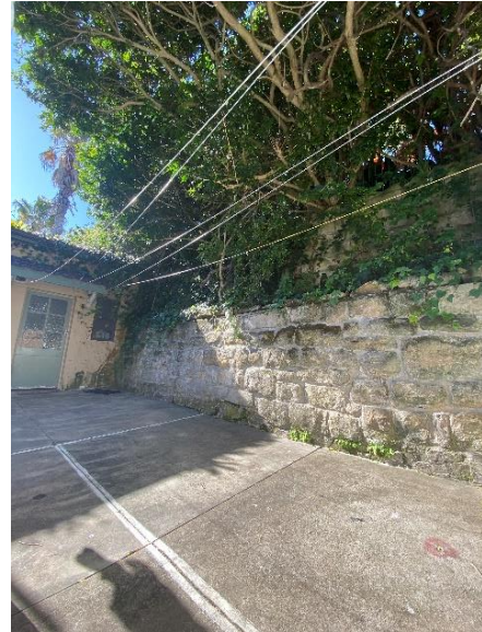
Figure 6: Existing rock wall along eastern (rear) boundary
