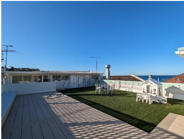
Figure 2: Existing roof-top balcony and roof additions, looking north-east
