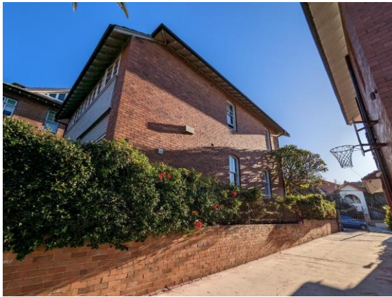
Figure 9: Northern side elevation of 14 Imperial Avenue viewed from rear driveway of subject site, looking south-west
