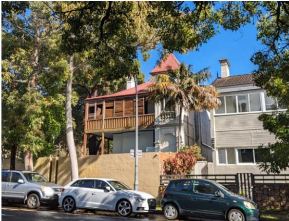
Figure 1: Site viewed from Flood Street, looking west
