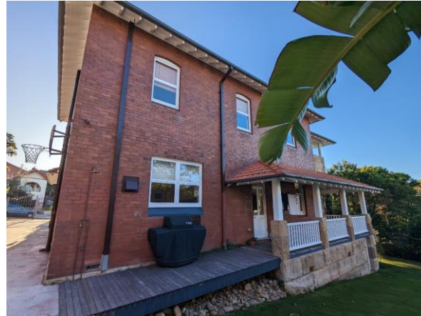
Figure 4: Rear of existing dwelling viewed from rear driveway, looking west
