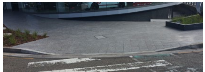
Pedestrian ramp pattern A, Bondi Junction
