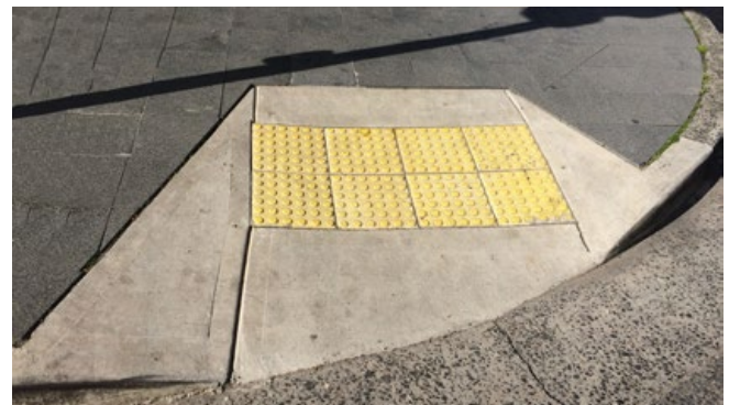
Pedestrian ramp pattern B, Bondi Road
