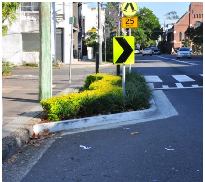
Integrated kerb extension- Ebley Street, Bondi Junction
