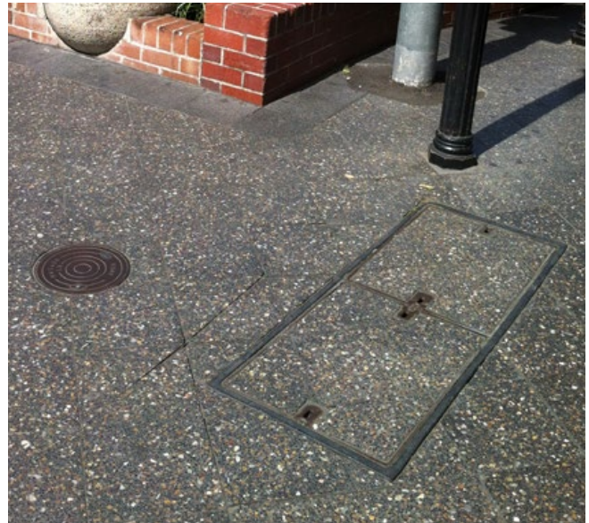
Service pit infill Bondi Junction
