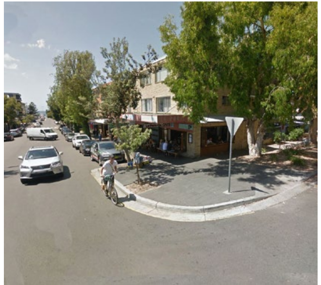
Integrated kerb extension- Hall Street, Bondi
