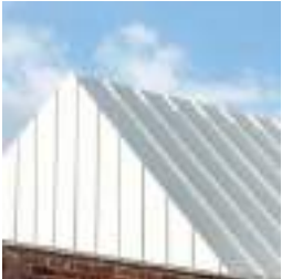
METAL ROOFING EuroPlus STANDING SEAM WITH CONCEALED FIXINGS SEVERE MARINE ENVIRONMENT FINISH COLOUR: SURFMIST / OFFWHITE
