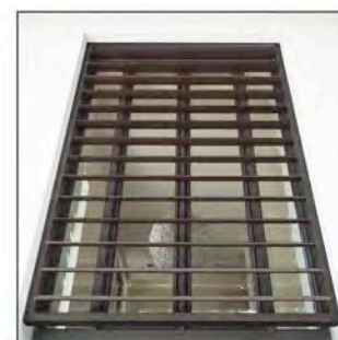
4. MOTORISED ALUMINIUM LOUVRES: LOUVRETEC 300mm AIRFOIL MAXI LOUVRE, POWDERCOAT, COLOUR DULUX "WOODLAND GREY"
