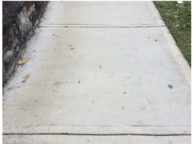
Concrete footpaths broom finish
