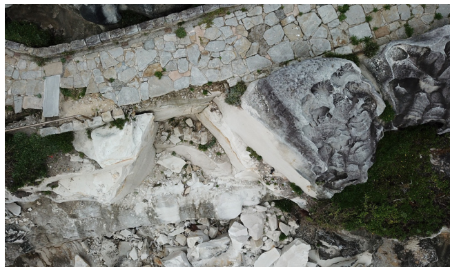
Coastal walk repairs beneath Marks Park
