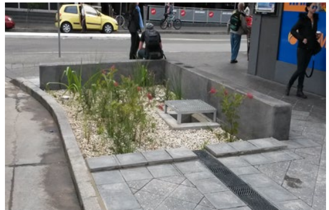
Bioretention Raingarden at Gray Street North
