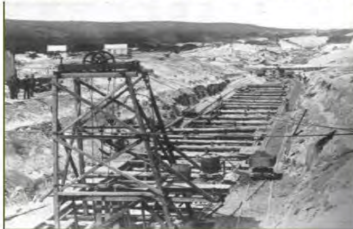
Figure 2.16: This section of the Bondi Ocean Outfall Sewer was oviform and brick lined (Water NSW)
