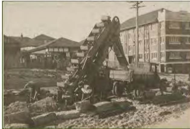
Figure 2.17: 'Barber Greene' excavator in operation on Campbell Parade, North Bondi. This undated image gives an idea of the types and depths of disturbance of the uppermost sandy soil profiles that are currently sealed below the current alignment of Campbell Parade (Waverley Image Library)
