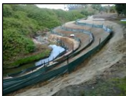
Weed control, bank stabilisation and resotoration of degraded and eroding creek in Penrith
