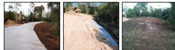
Sandstone capping of land contaminated by Asbestos
