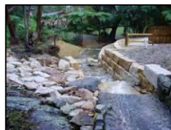
Sandstone retaining walls as recommended for Zone 2
