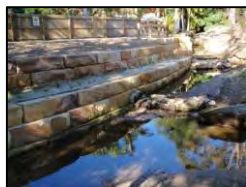
Sandstone retaining walls as recommended for Zone 2
