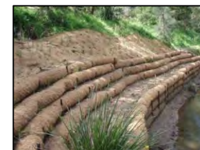
Restored creek bank w/ coir logs
