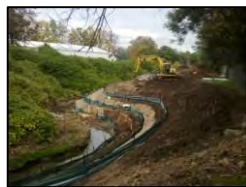
Weed control, bank stabilisation and resotoration of degraded and eroding creek in Penrith
