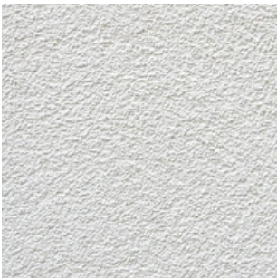
RN1 - CEMENT RENDER. APPLIED TO ALL EXISTING WALLS. NEW RENDER TO MATCH.
