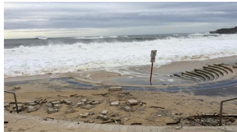
Figure 3-5 Coogee Promenade damaged during the 2016 storm (Source: Daily Telegraph, 2016)
