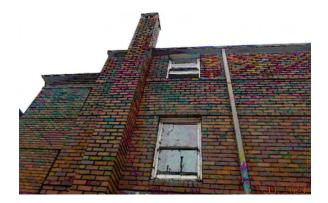
EXISTING FACE BRICKWORK Existing face brickwork with string courses and shaped sill bricks to be retained and repointed as required. New brickwork to be from carefully recycled from on site demolition
