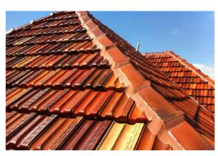
EXISTING ROOF TILES Terracotta roof tiles to be replaced as required with similar to match existing
