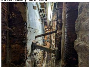
**Figure 9:** Excavated drainage channel located adjacent to the western boundary of 9 Thompson Street toward the central and norther part of that site, viewed from 9 Thompson Street looking north. The boundary retaining wall with 7 Thompson Street is at the left of the photo. Thompson Street features numerous garages or other structures built with nil setbacks to side boundaries, including at numbers 9, 11, 15 and 23, and a recent approval at number 27.
