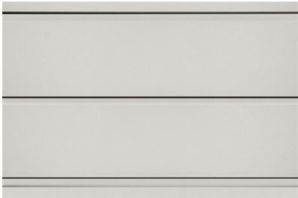
HORIZONTAL WEATHERBOARD CLADDING TO EXISTING FIRST FLOOR EXTENSION, PAINTED WHITE, ALUMINIUM WINDOWS POWDERCOAT
