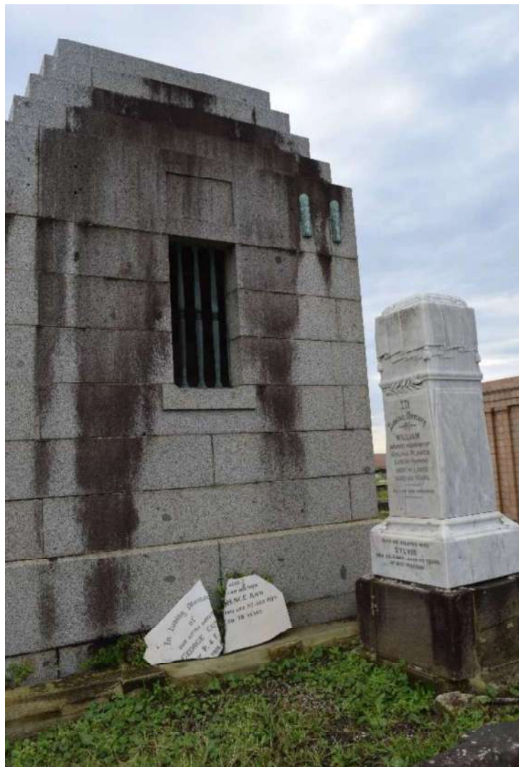
Dirt created to vault façade through by water run-off.
