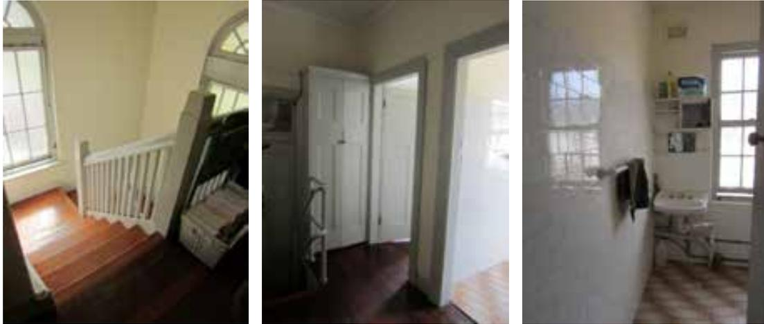
Figure 120 The first floor of the Auditorium pavilion has retained a substantial amount of original fabric including its stair (left; F28), doors, a cupboard, skirting boards and picture rails (centre; F27). However, the bathroom has been refurbished (right; F24).
