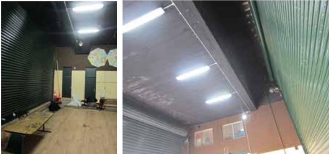
Figure 118 Stage area within the early 1930s Auditorium pavilion. The former caretaker's residence above, now used for office purposes, only extends over part of this space and has a reinforced concrete floor slab supported off a deep reinforced concrete beam.
