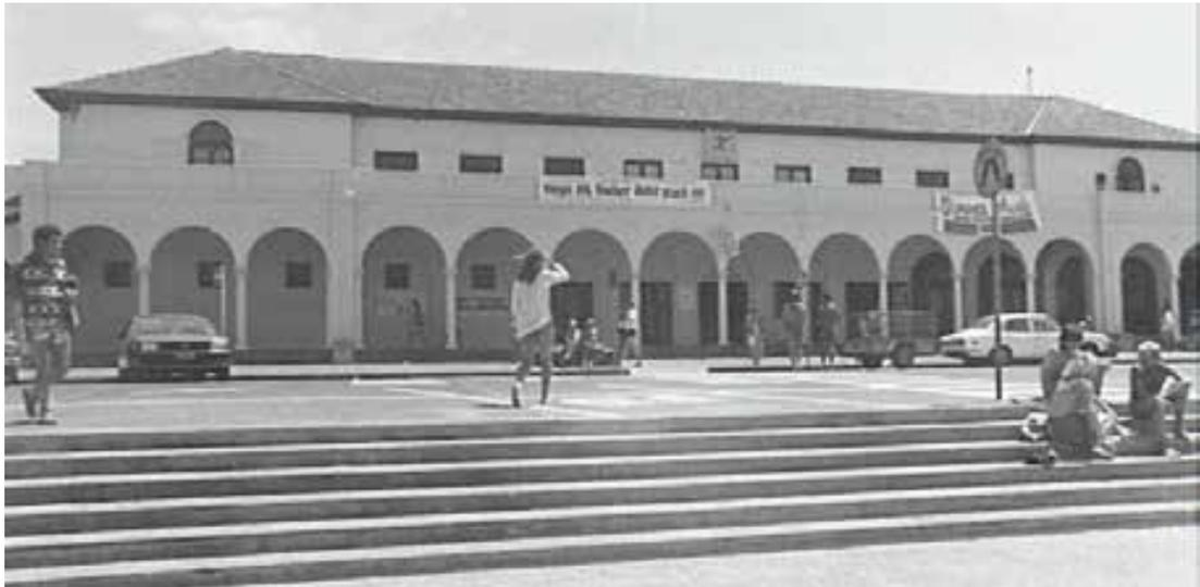
Figure 78 This 1980 photograph shows the configuration of original fenestration associated with the Turkish Bath on the western side of the principal facade and the door openings associated with retail tenancies on its eastern side. The recent arched openings in the western section of the elevation have been undertaken in a sympathetic manner, echoing the openings associated with the eastern retail spaces that already existed.
