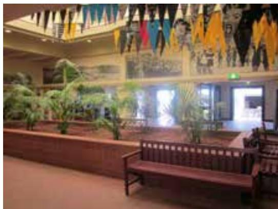
Figure 99 The former bathing costume/towel hire area and light well have been modified and opened up on its eastern side to become an atrium. The well-intentioned brick planter is an inappropriate element within the space. Interpretive photographs have been mounted around the space. Quarry tiles covering the floor are not original.
