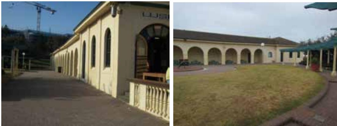
Figure 82 Looking north along the western facade. The balustrade has been modified to provide access to the tenancy space that now occupies the shower room (left). The western facade incorporates a secluded loggia (right).
