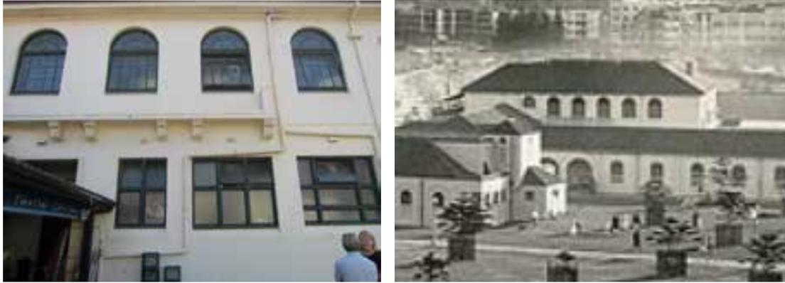
Figure 93 Evidence of a removed balconette. The absence of a sill moulding at the base of the three windows above the remnant balconette suggests that these may once have been door openings. The archival photograph indicates the presence of the balconette during the 1930s.
