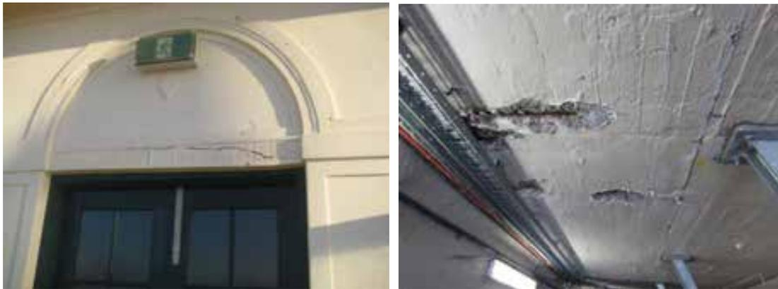
Figure 156 Cracking in rendered wall surface above a first floor door opening on the southern side of the Pavilion (left) and exposed reinforcement in the soffit of a groyne tunnel (right).
