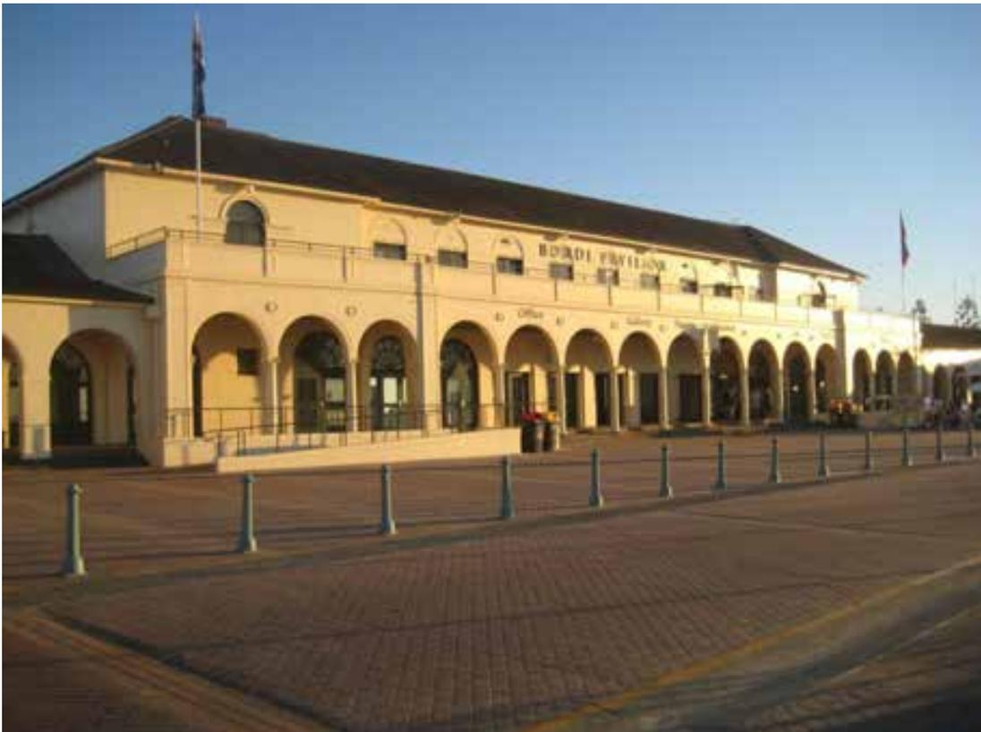
Figure 77 Principal elevation of the Bondi Pavilion in March 2015. Modifications include ramps, arched openings in the western section of the elevation, addition of signage above first floor windows, ramps and the handrail above the balcony balustrade wall coping. Signage mounted on wall surfaces is also relatively recent.
