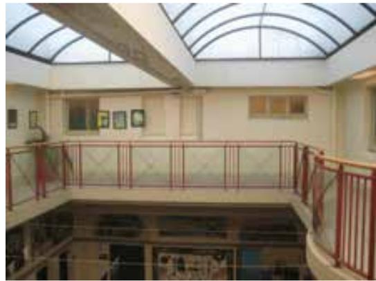
Figure 109 Upper level of the Atrium (F10), originally a light court and modified by the construction of a perimeter mezzanine and enclosed by translucent vaults.
