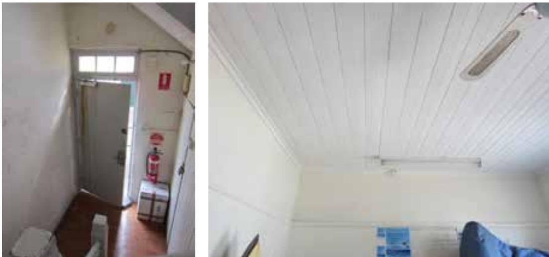
Figure 119 Ground floor vestibule associated with the stair to the former caretaker's flat (left, G45). The first floor spaces largely have timber board lined ceilings (right), although some have battened sheet linings, possibly of fibrous plaster.
