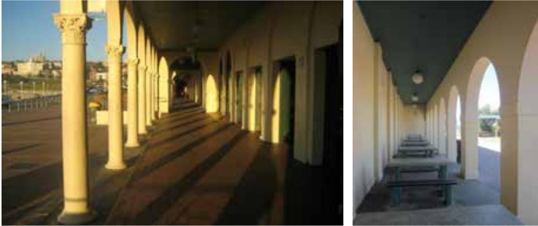
Figure 86 Views along the southern loggia (left) and western loggia with 1930s tables and benches (right). Early photographs show the floor of the southern loggia was originally concrete. The original margin beneath the columns has been retained. Loggias generally have retained timber soffit linings.
