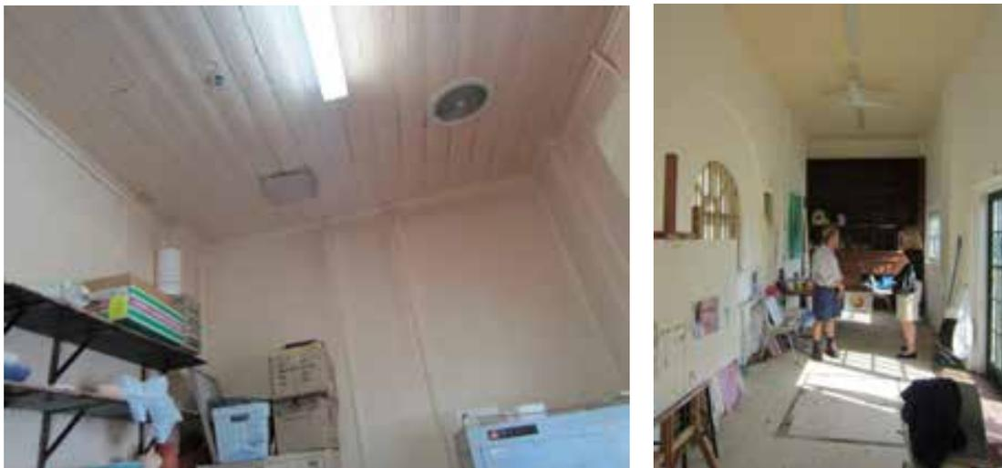
Figure 104 Although the spaces occupied by the craft studios (G4 and G5) are located in former lavatories and loggias, original fabric including timber ceiling linings, has been retained.
