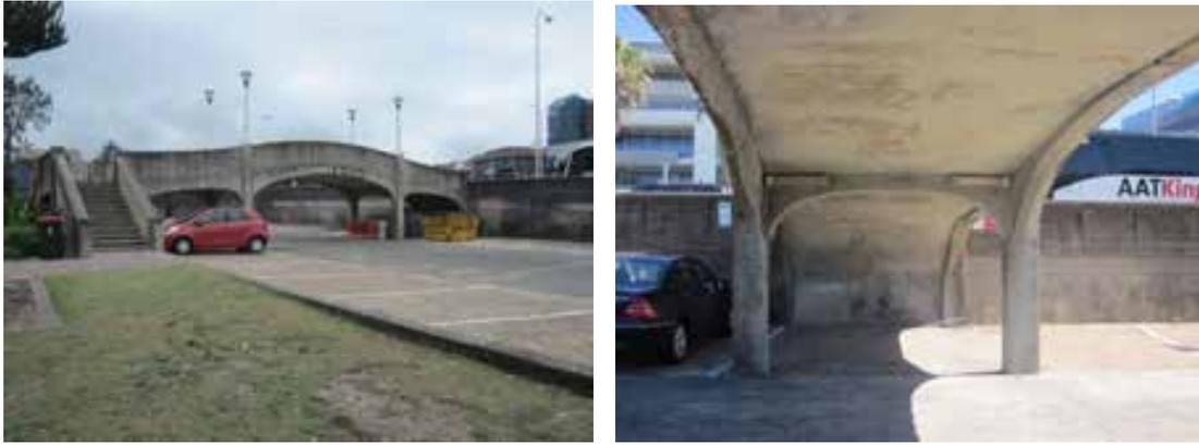
Figure 137 The form of the pedestrian bridges is typical of this period when compared to similar structures such as the bridge at Balmoral Beach. The reinforced concrete fabric of the bridges is in good condition.
