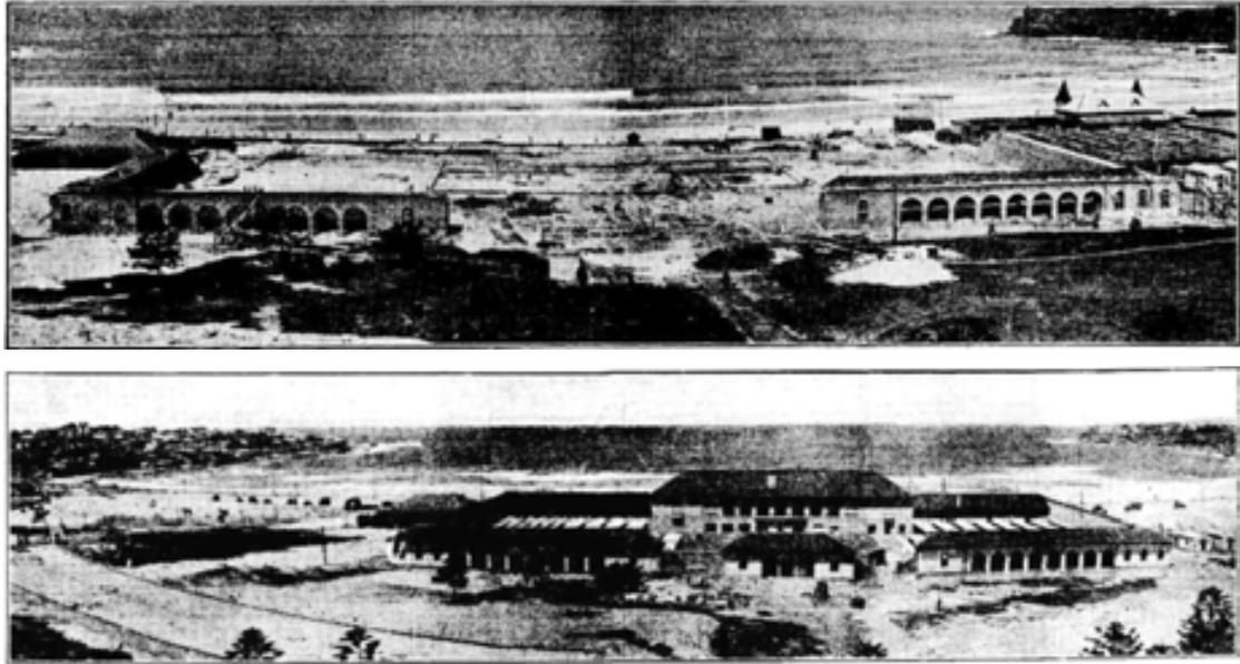
Figure 19 The Bondi Pavilion under construction in April 1928 (top). The relocated 1916 surf club house can be seen at far left, the 1911 surf pavilion at far right. Six months later the “new Casino and Surf Pavilion” had progressed rapidly (below).
