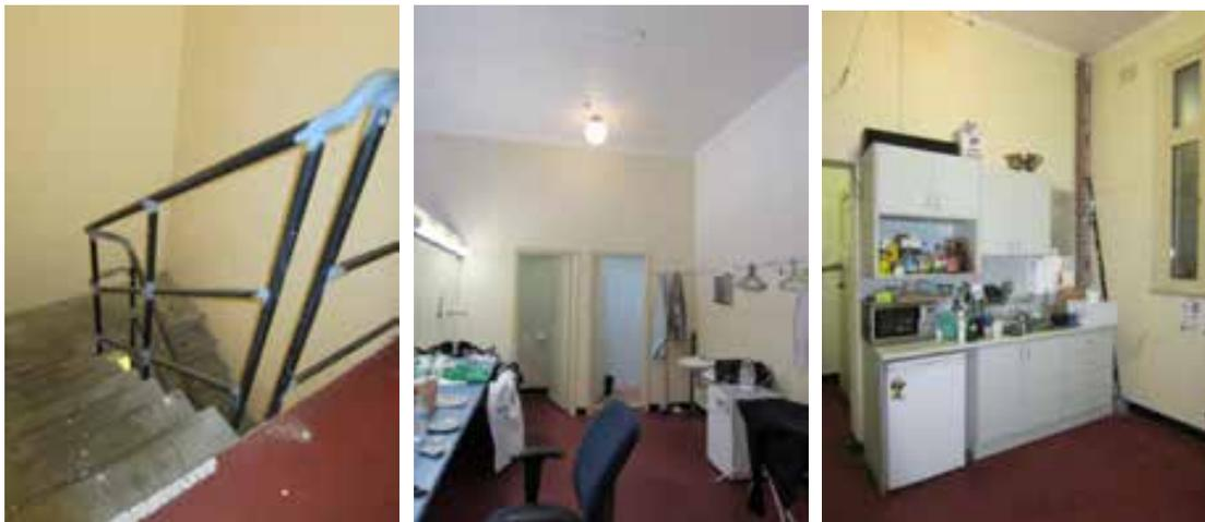
Figure 115 Escape stair (F16) and ancillary rooms associated with the Theatre, located in the space originally occupied by the dining room kitchen (F19-F21). The ceilings, as with many other spaces within the Bondi Pavilion, are lined with timber boards.
