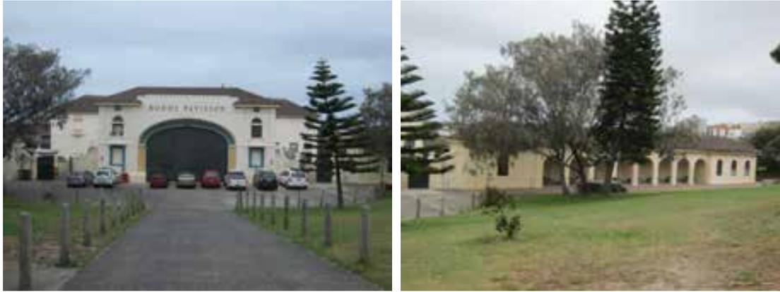
Figure 83 The central two storey pavilion on the northern side of the building is dominated by the large arch that formed the proscenium for the stage of the outdoor auditorium. The single storey wings on either side of the pavilion have retained original arcaded loggias (right).
