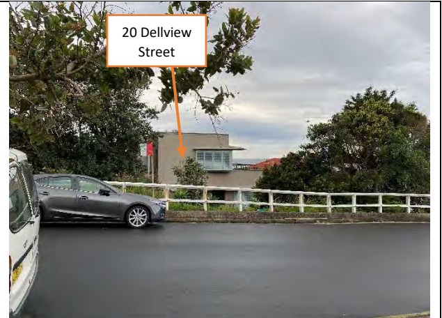
Figure 2: View across Dellview street.
