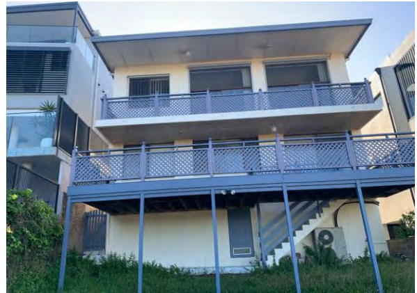
Figure 2: Easterly view of the rear façade of the dwelling.
