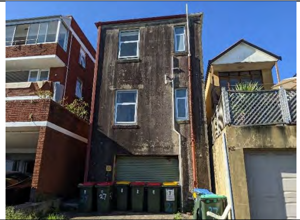
Figure 2: Site viewed from Dellview Lane, looking north
