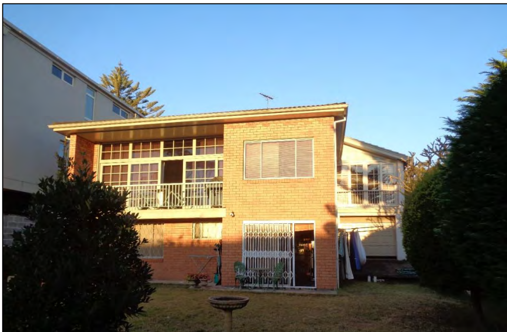
Figure 2: Rear elevation of existing dwelling
