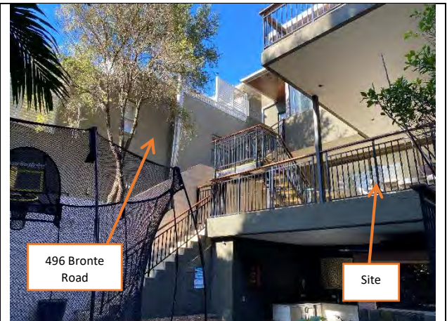
Figure 8: Rear view of 496 Bronte Road
