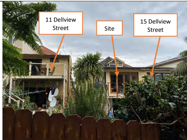
Figure 3: Rear view of the subject site.
