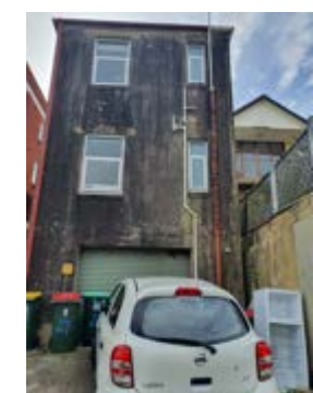
R REAR OF SUBJECT SITE SHOWING ADJACENT No. 25 FLETCHER ST.
