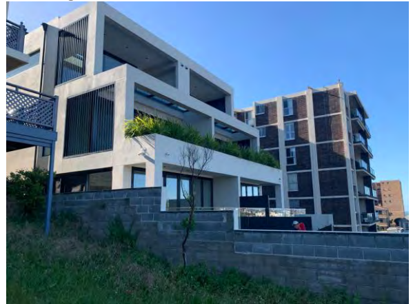
Figure 4: Southerly view of the neighbouring dual occupancy and apartment building at 58 and 56 Military Road.
