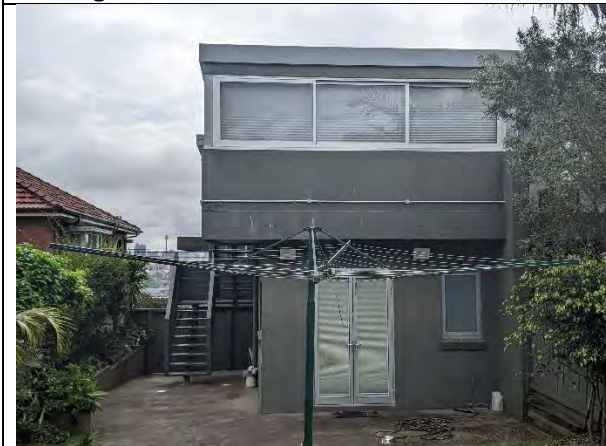
Figure 3: Site viewed from rear yard, looking west
