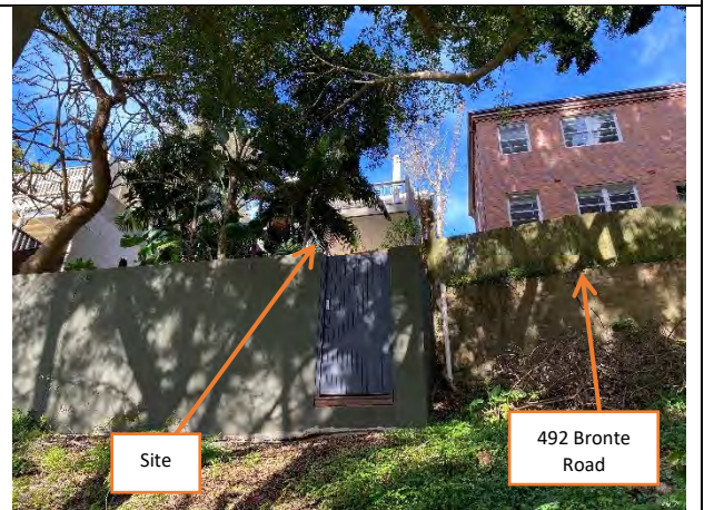
Figure 4: Rear view of the subject site from Bronte Park
