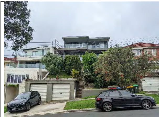
Figure 1: Site viewed from Gilbert Street, looking east
