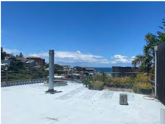
Figure 5: Existing roof facing east
