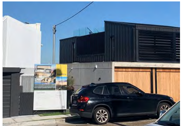
Figure 6: Westerly view of the existing roof terrace at 64 Military Road.
