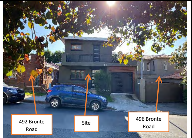
Figure 2: Streetscape view of the subject site.
