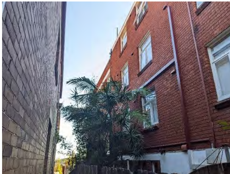
Figure 3: View from western side setback, looking south. The subject building is at the left of the photo, and 25 Fletcher Street is at the right of the photo
