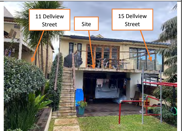
Figure 4: Rear view of the subject site.
