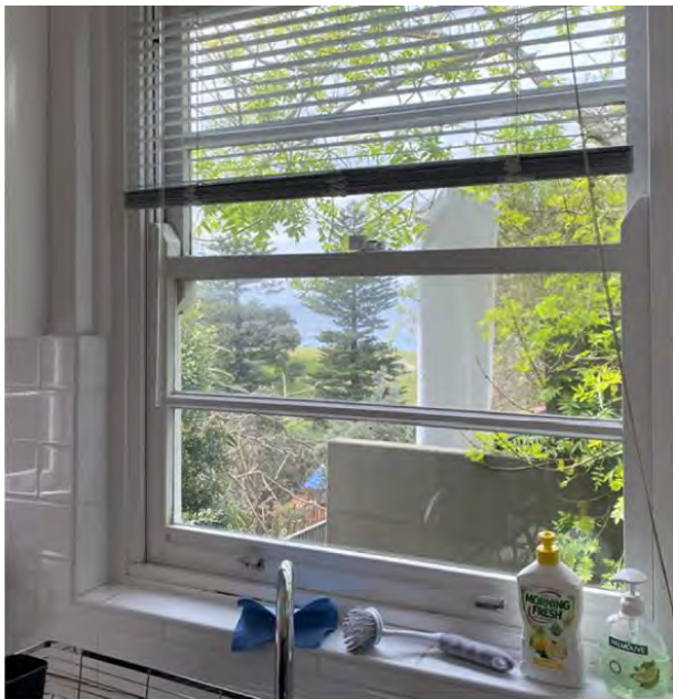
VIEW 1 - GROUND FLOOR KITCHEN WINDOW - EXISTING
