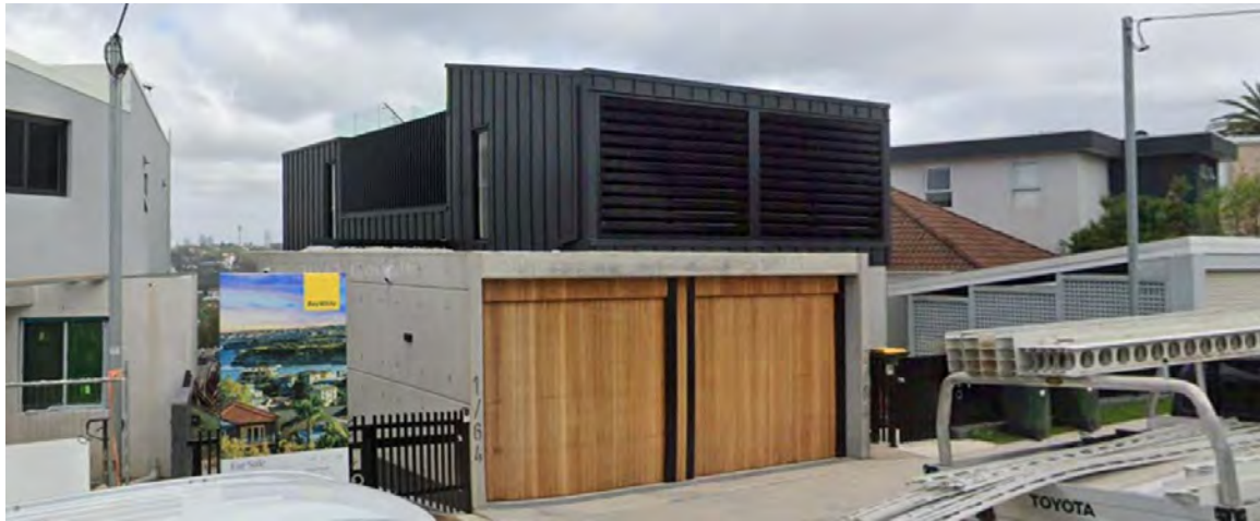
Figure 10: Recently approved and completed roof top terrace at 64 Military Road, 2 properties to the north.
