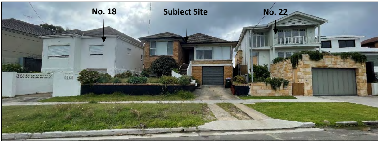
Figure 1: Subject site as viewed from Wentworth Street (Source: Google Maps, 2023).
