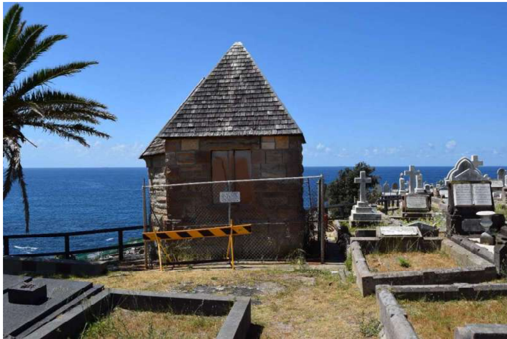
Figure 129: A small sandstone structure with steep timber-shingled roof is located on the eastern boundary of Section 17. It is currently inaccessible due to the recent landslip. View facing east.
