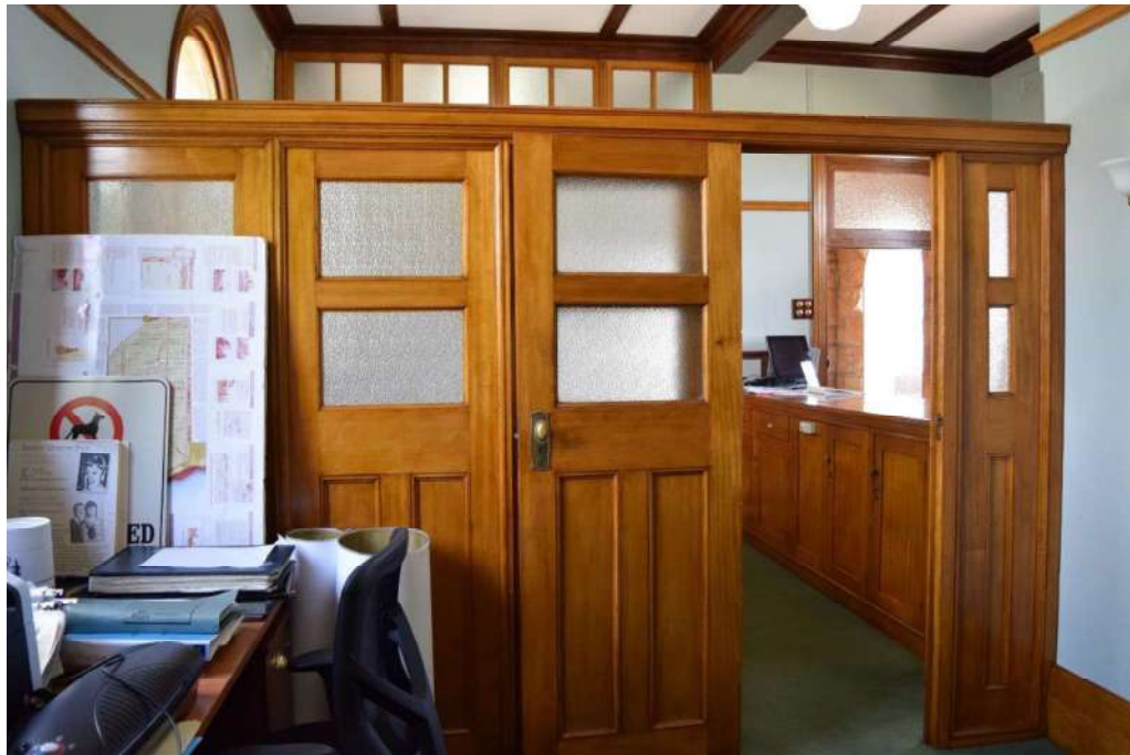
Figure 33: The interior of the office is one large space, divided by half height glazed timber partitions. The ceiling features timber coverstrips and timber picture rails are present on the walls. Interior furnishings are a more recent addition.
