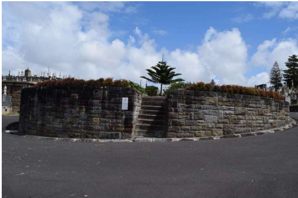
Figure 63: The sandstone random ashlar retaining wall which contains a raised rondel garden with radially-arranged ash interments.
