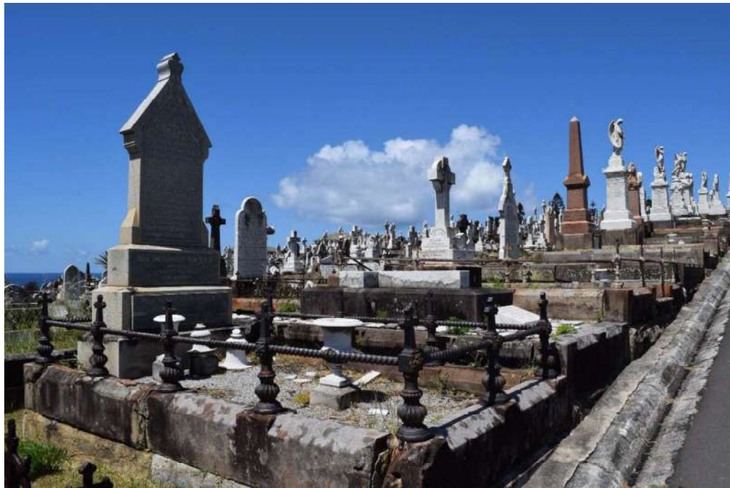
Figure 127: Cast iron surrounds on graves is clearly corroded as the result of rust and exposure to sea spray. This damp is also manifest in the lichens and on grave surrounds. View facing south-east.
