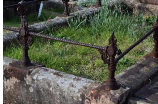
Figure 156: Corroded metal caused by deposition of salts by sea breezes
