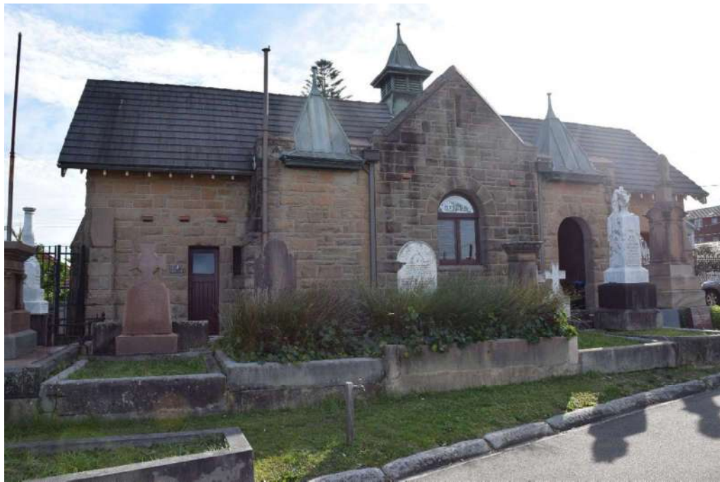
Figure 31: Eastern elevation of the Cemetery Office with steep pitched gabled roof and smaller, decorative pyramidal roofs clad in metal.
