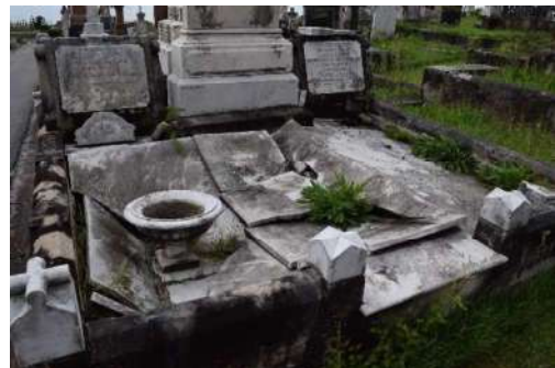
Figure 158: Fracture of a grave covering caused by subsidence of the ground.
