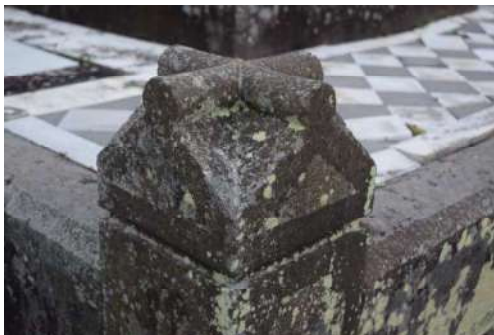
Figure 157: Stone monument damaged by lichen growth.
