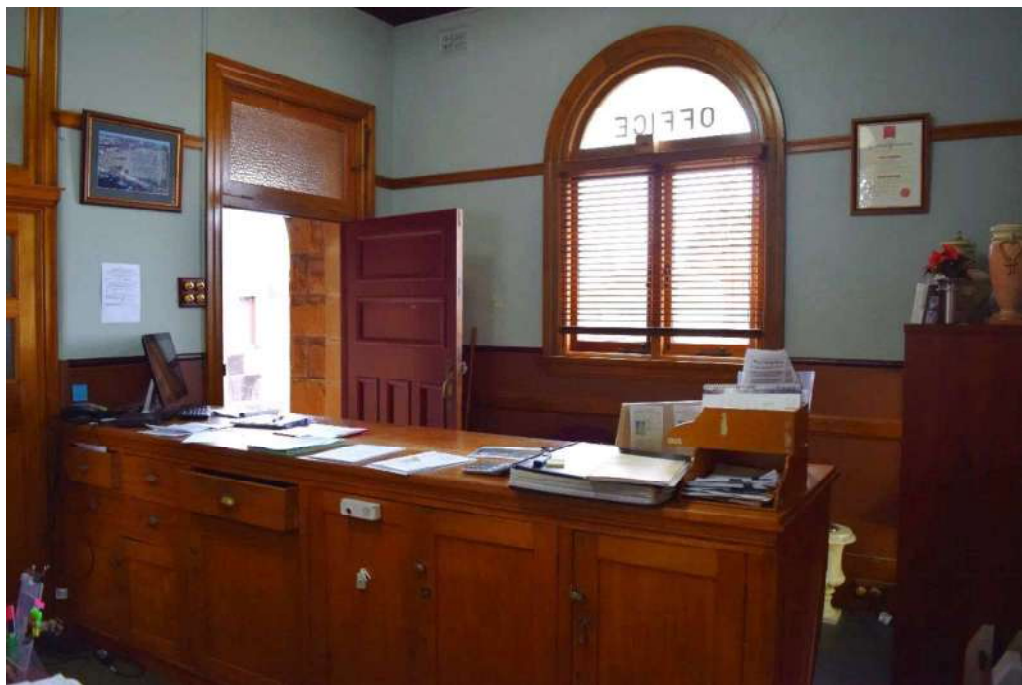
Figure 35: The main Cemetery Office reception desk. Note the timber dado and picture rail, fanlight above the main entrance door and the half round window opening.
