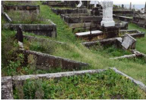
Figure 159: Graves and stone surrounds that have sunk due to subsidence of the ground.
