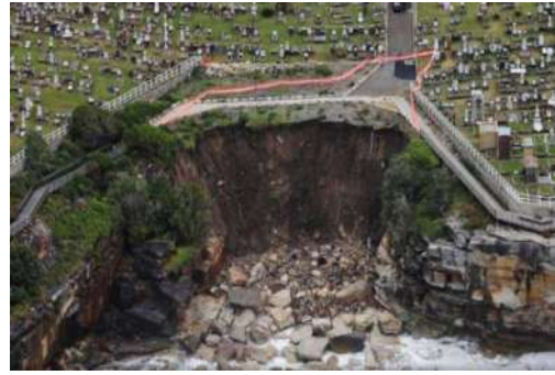
Figure 160: Landslip following the 2016 destructive coastal storm. (Source: Waverley Council)
