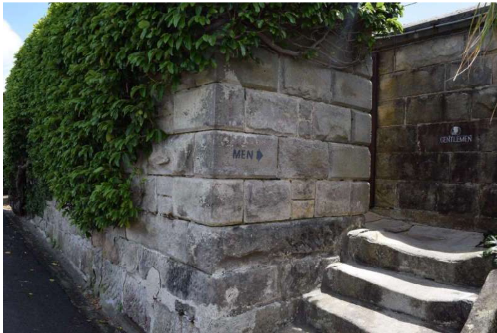
Figure 46: Sandstone wall and steps to the men's toilet. Note tree to the west has extended over the wall.
