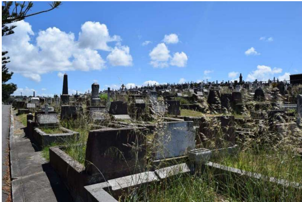
Figure 151: Like Section 20, graves in Section 21 are full of vegetation, particularly weeds, and are hollowed from subsidence and erosion. View facing north.
