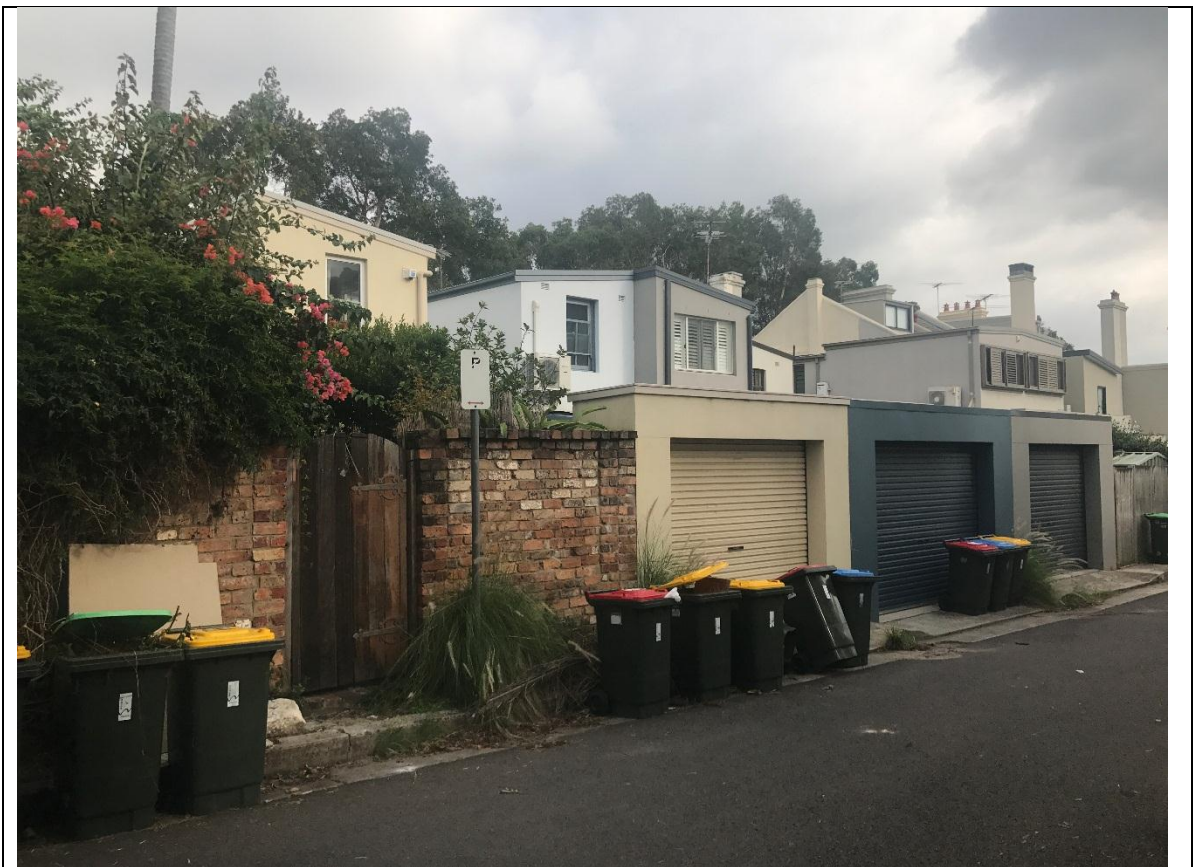
Figure 5: Rear of terrace row viewed from Gowrie Lane
