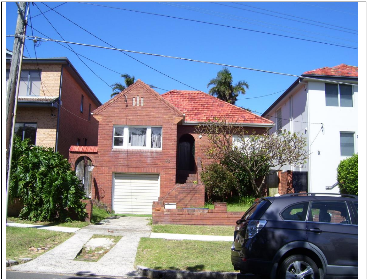
Figure 1: Site as viewed from Hardy Street (an elevated single storey red brick dwelling with garage below at centre)
