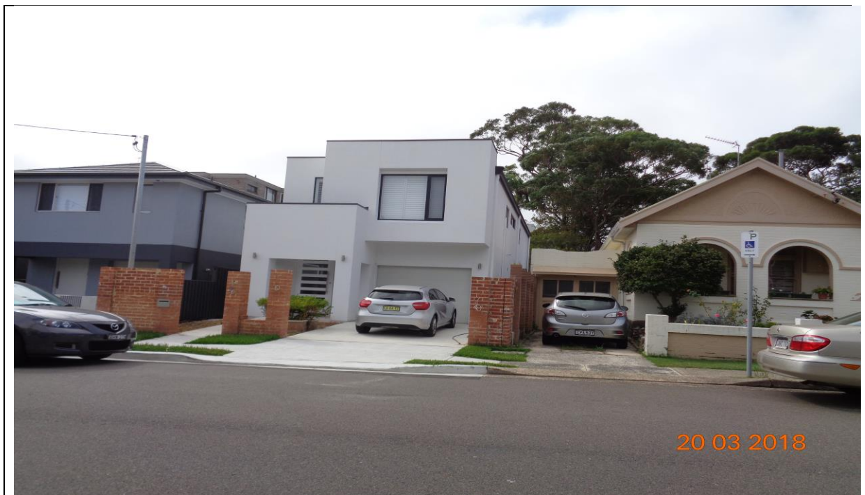
Figure 1: Subject site. (Fence structure built contrary to condition 2 (a) of DA-181/2017)
