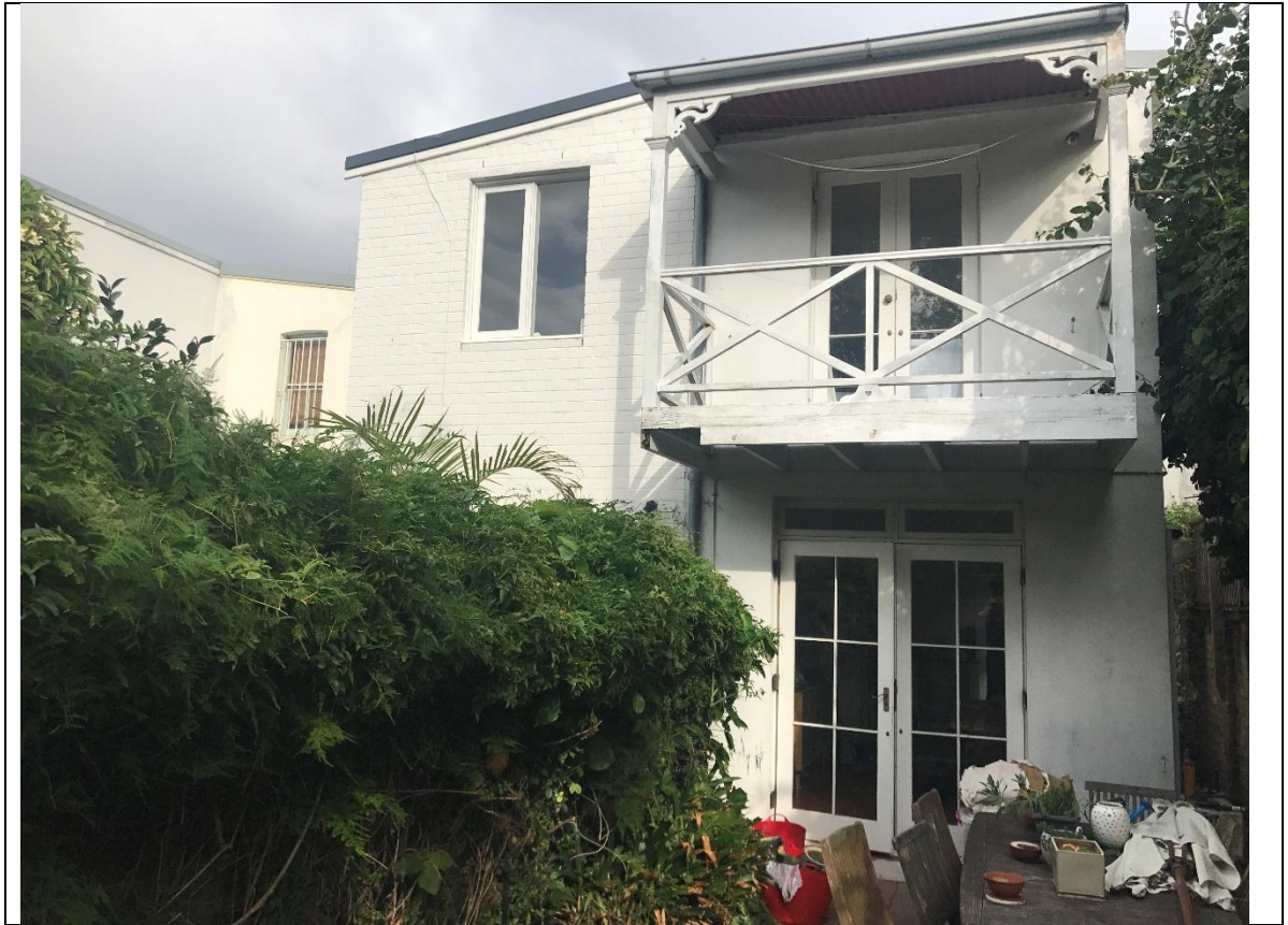
Figure 2: Rear of site and neighbouring terrace at 30 Ruthven Street
