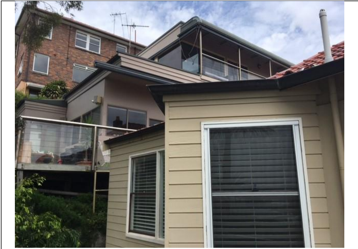
Figure 2: Subject site viewed from the rear neighbouring balcony of No.44 Gardyne Street
