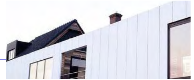
CT3 - WHITE COMPOSITE PANEL CLADDING
