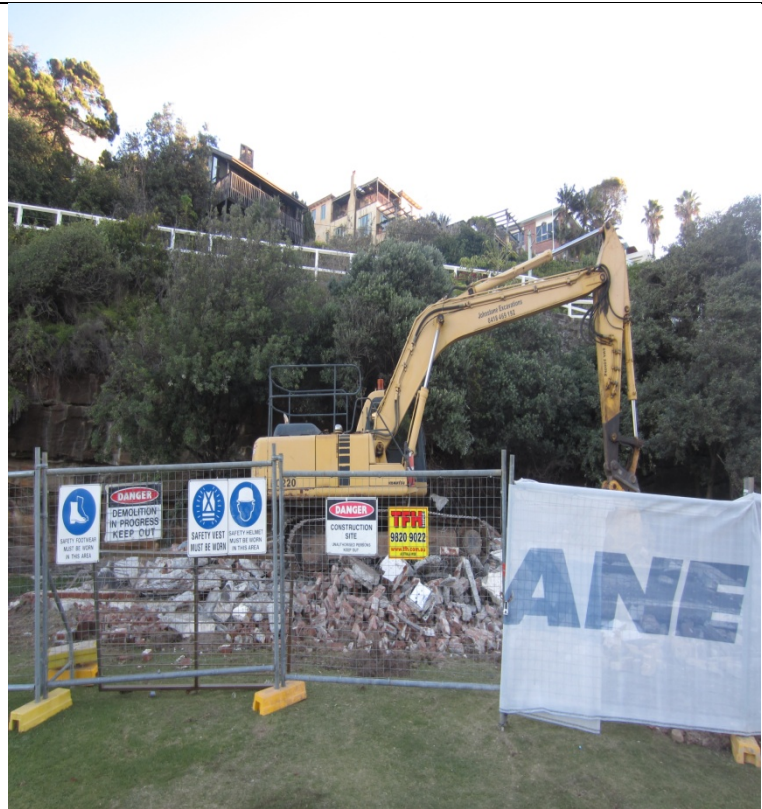
Tamarama Kiosk Building Demolition
