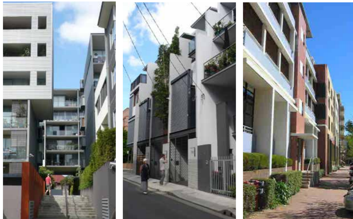
Figure 34 Photographs showing connections with new housing
