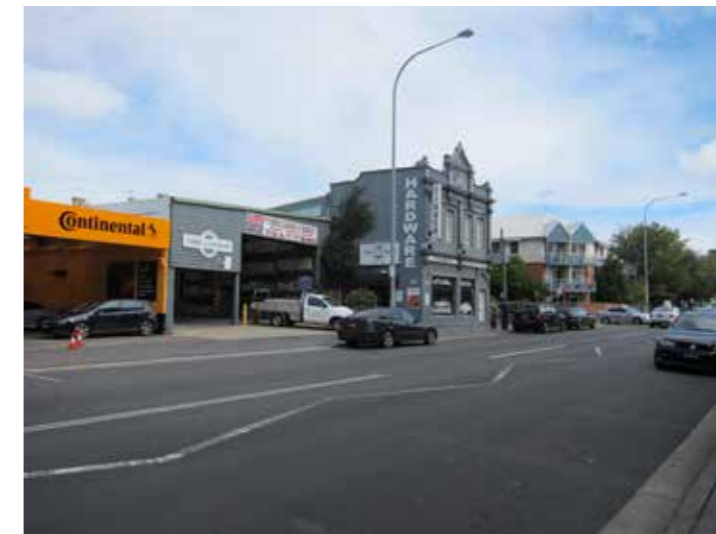
Figure 6 Timber and tyre yard between Denison Street and Mill Hill Road
