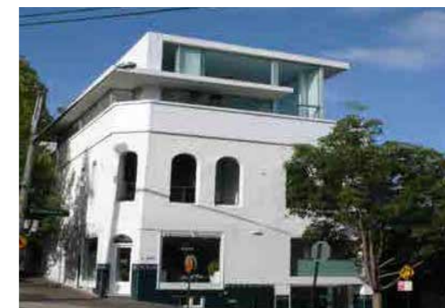
Figure 67 Add to older buildings
