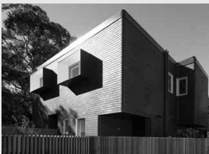
Design Award for Design Excellence for a Multiple Dwelling 23 Brown Street, Bronte 'Double House' Neeson Murcutt Architects
