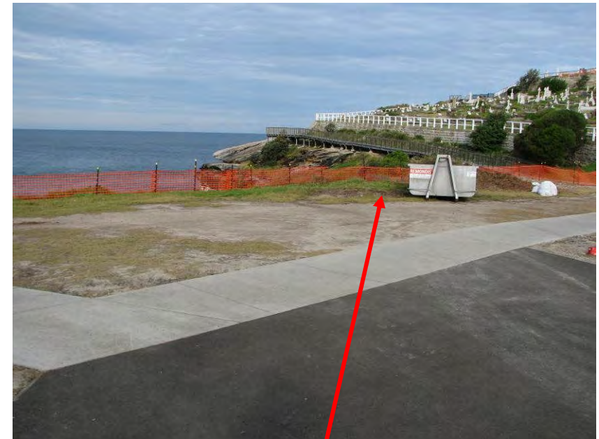
Crest area of gully feature
