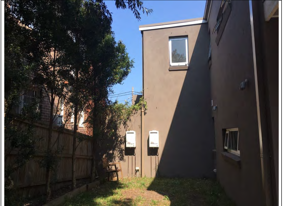
Figure 3: View from rear yard (location of proposed side addition)
