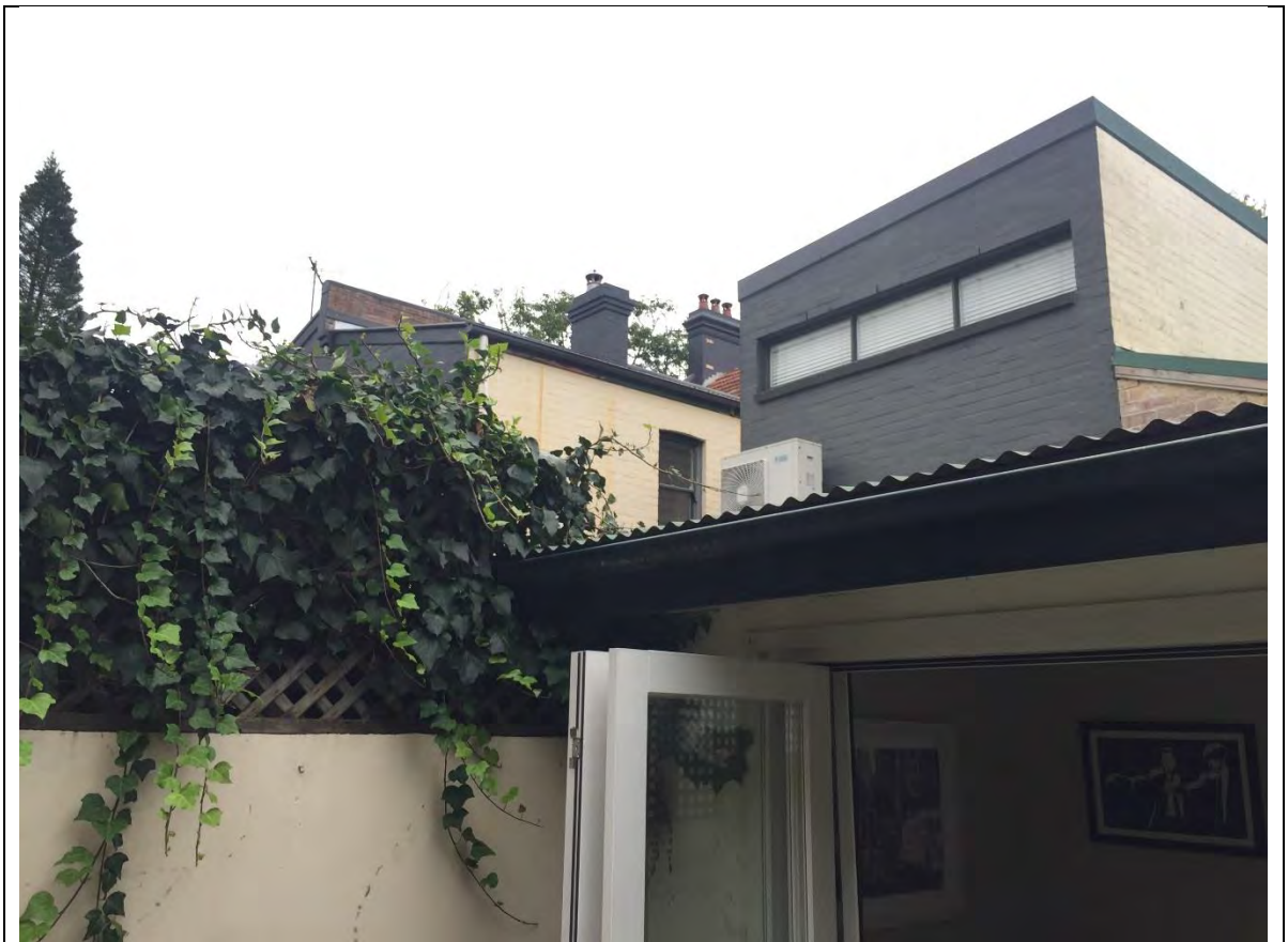
Figure 3: Rear view of 4 and 6 Watkins Street.
