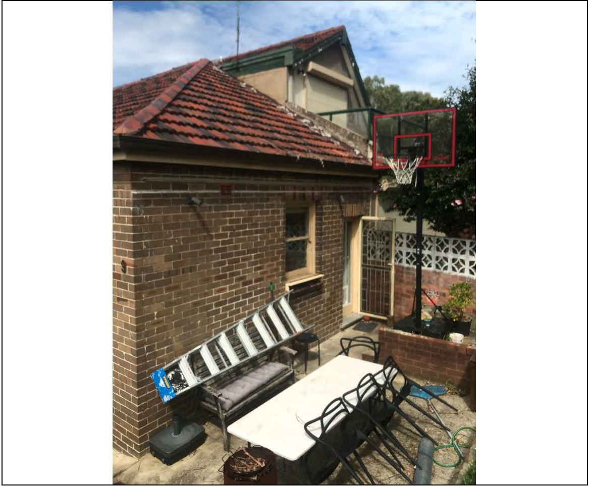
Figure 2: Existing rear elevation of the site
