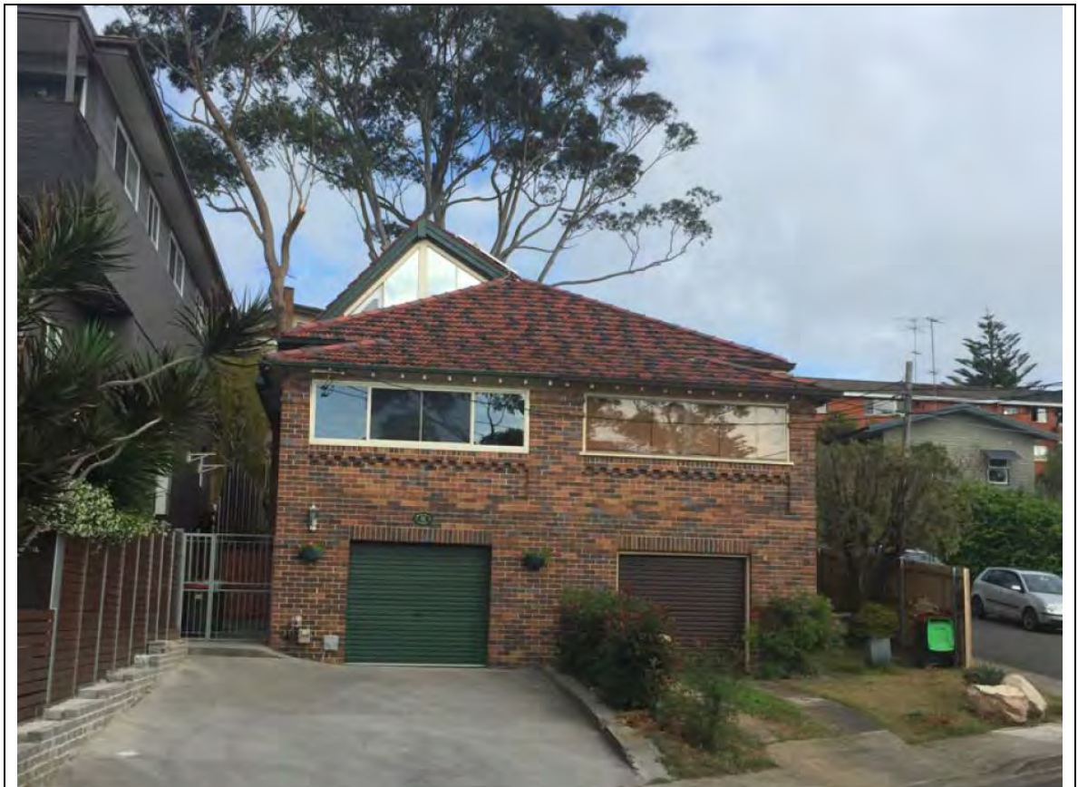
Figure 1: Site viewed from Wallace Street (number 9 is the dwelling on the right)
