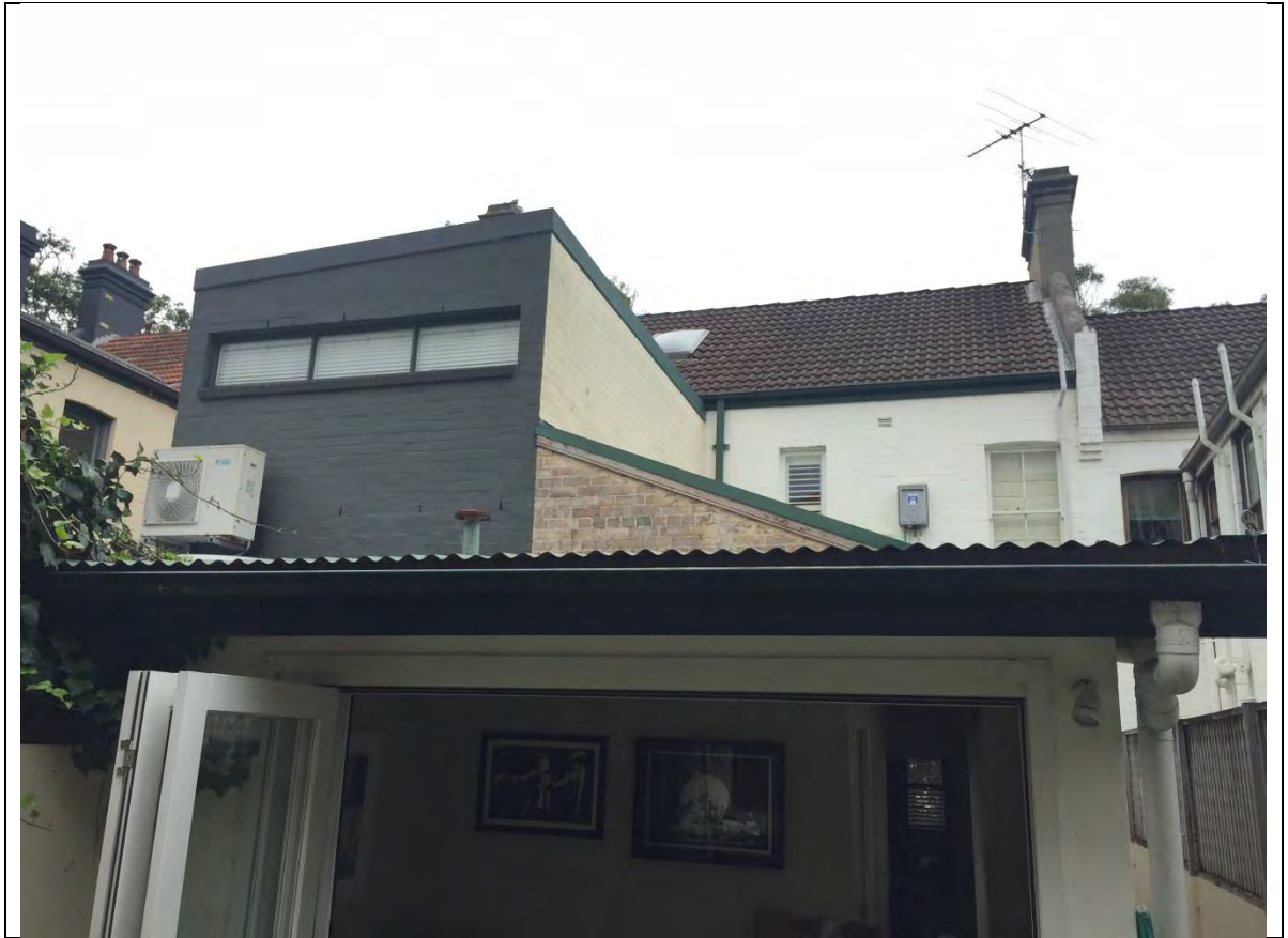
Figure 2: Rear view of 6 and 8 Watkins Street.
