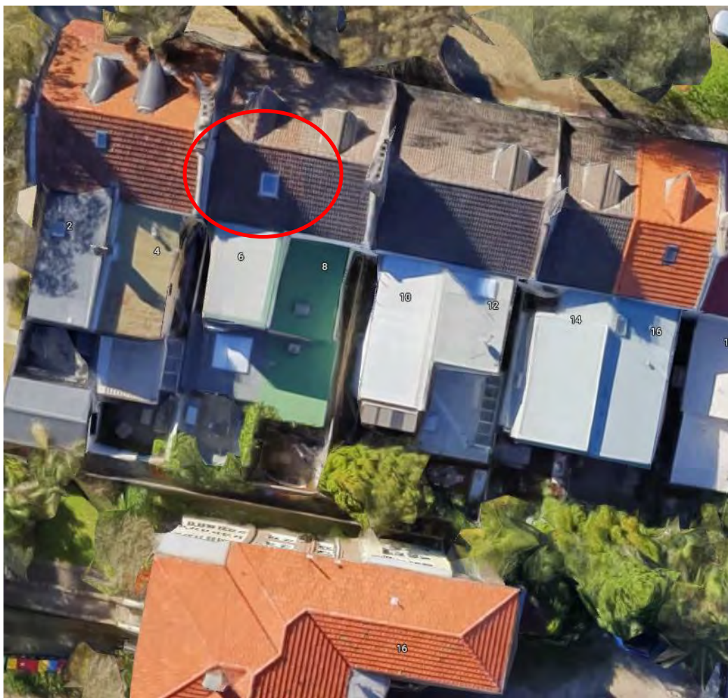
Figure 5: Extract from Google Imagery demonstrating the skylight at 6 Watkins St and existing overshadowing.
