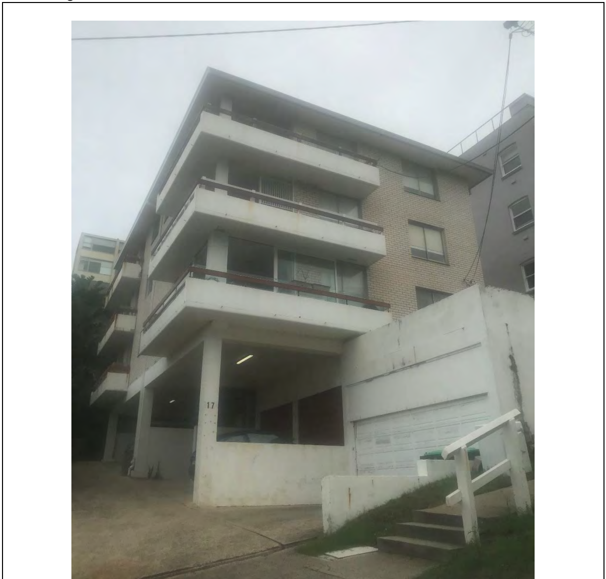
Figure 1: Subject site frontage
