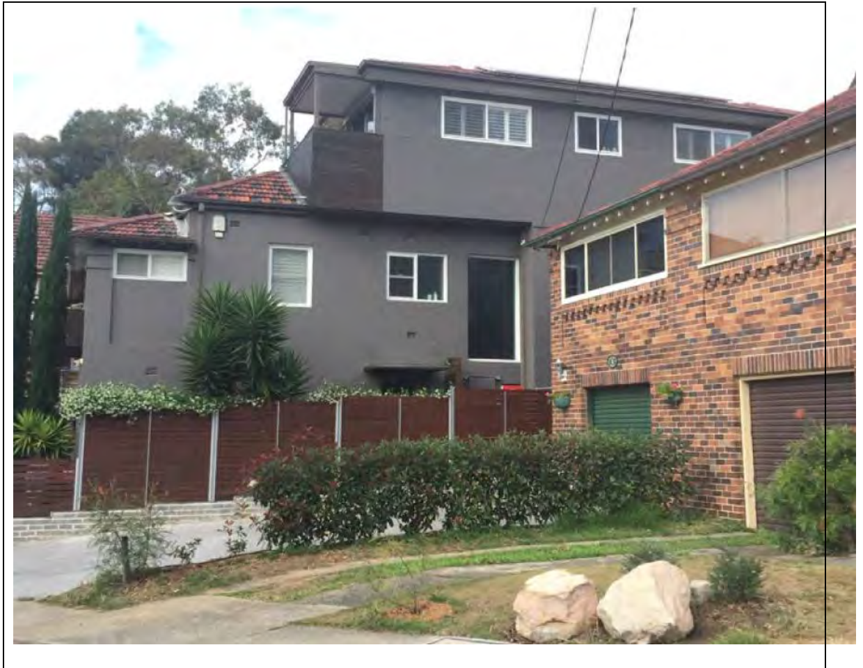
Figure 3: First floor addition at 13 Wallace Street
