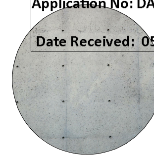
E - Off-form Concrete to Planterboxes
