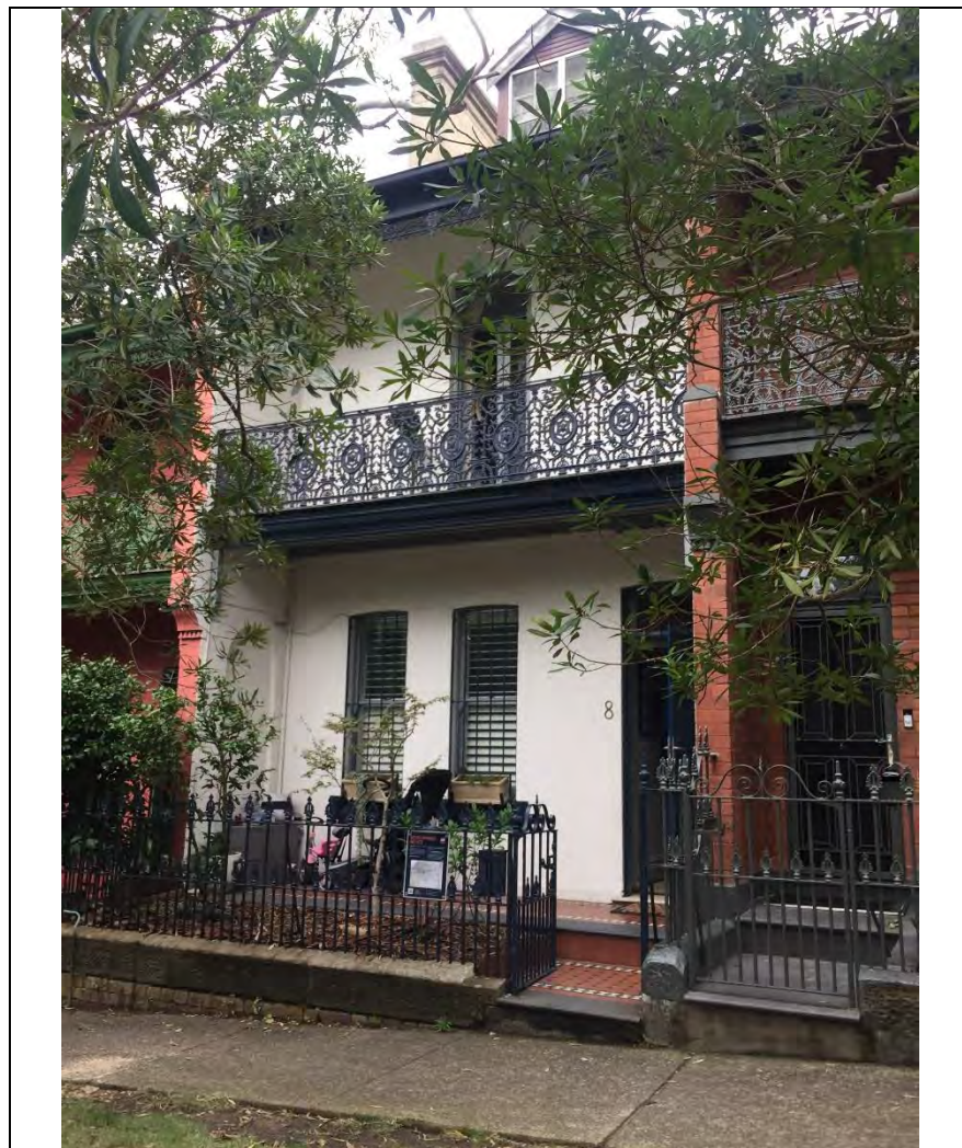
Figure 1: Subject site frontage
