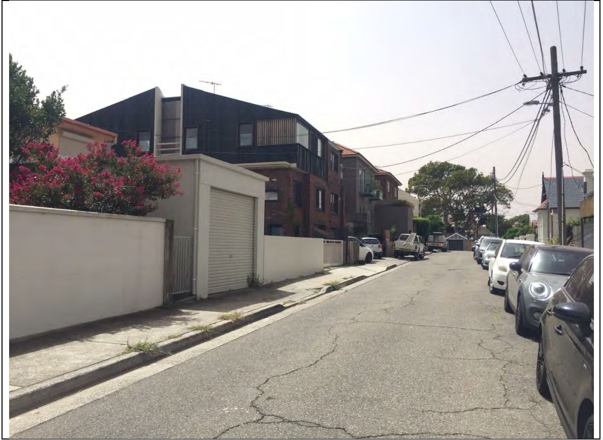
Figure 2: Streetscape of the northern side of Kent Street (2 to 10 Kent Street)
