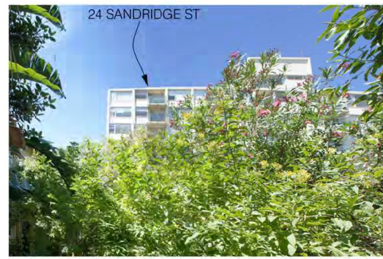
THE REAR OF 20 SANDRIDGE ST IS STEEP WITH LITTLE TO NO ACCESS TO THE STREET
