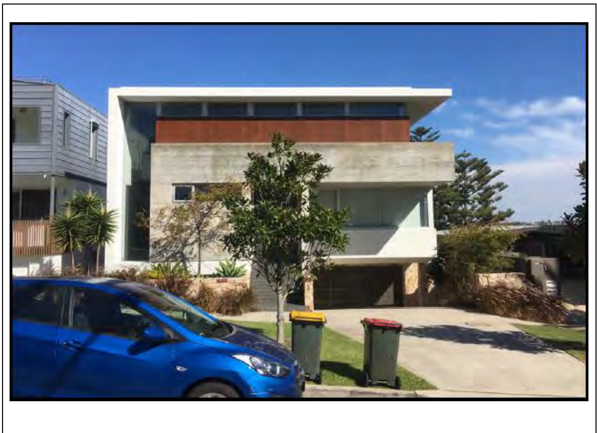
Figure 1: Site viewed from the street (Source – aSquareplanning)
