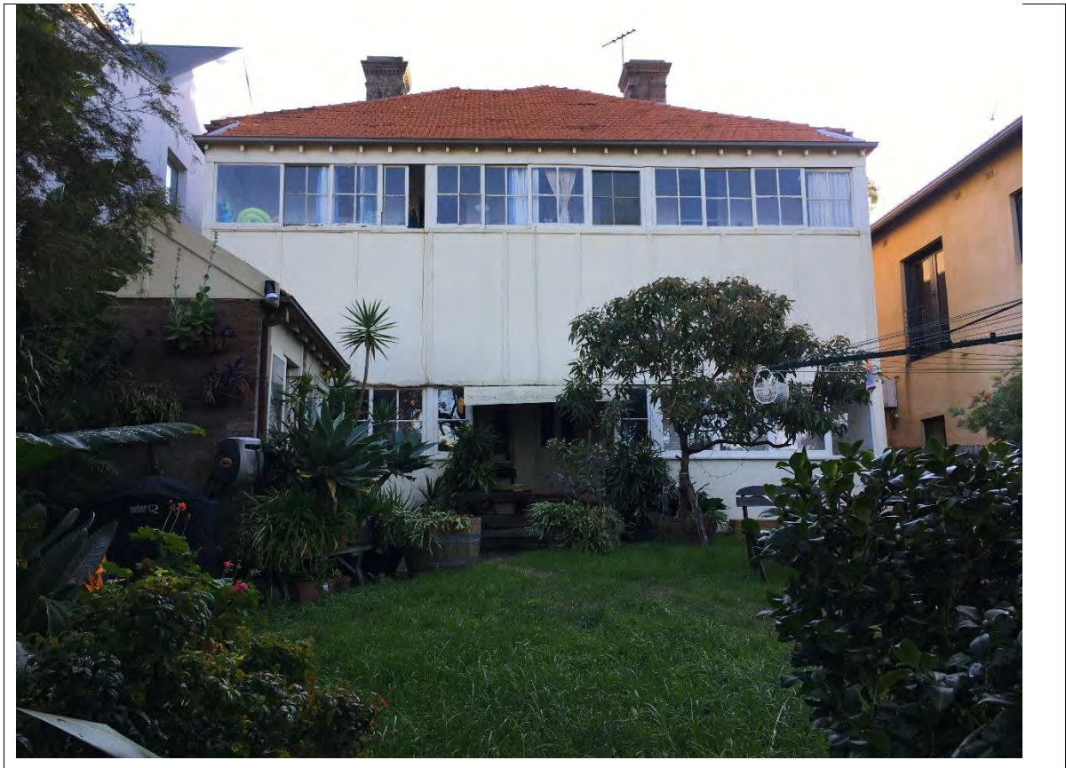
Figure 2: Existing building viewed from rear of the site
