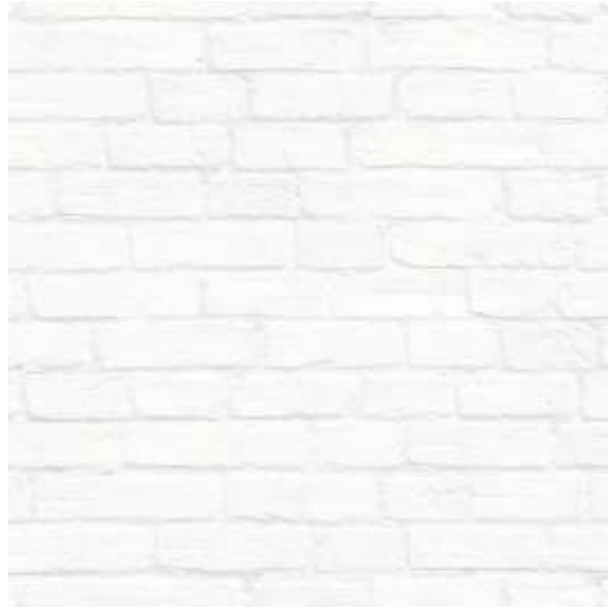
WHITE BAGGED BRICK: ALL EXTERNAL WALLS
