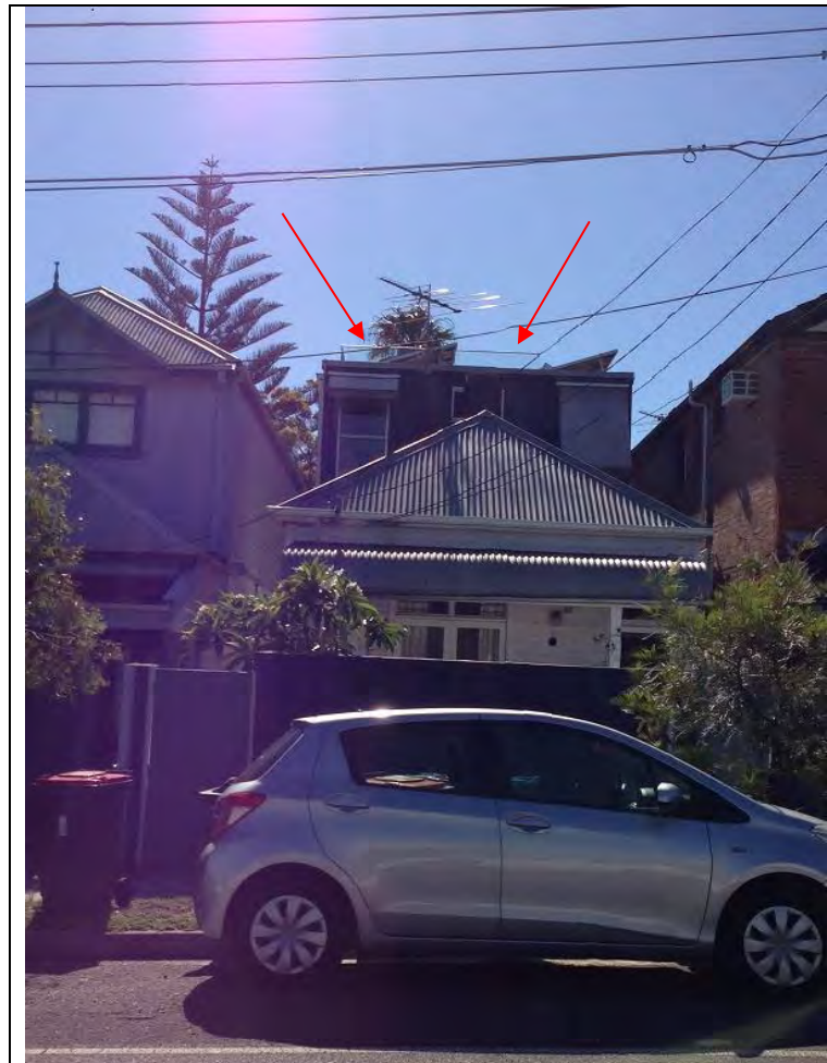
Figure 1: Subject site frontage (roof terrace balustrading visible from pedestrian view)
