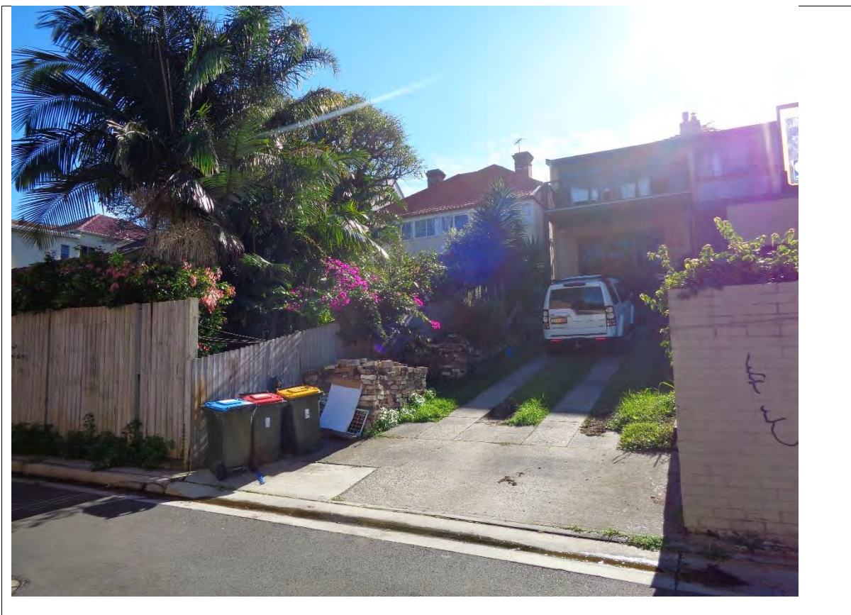
Figure 3: Site (with existing large tree) and neighbouring development viewed from Chesterfield Lane
