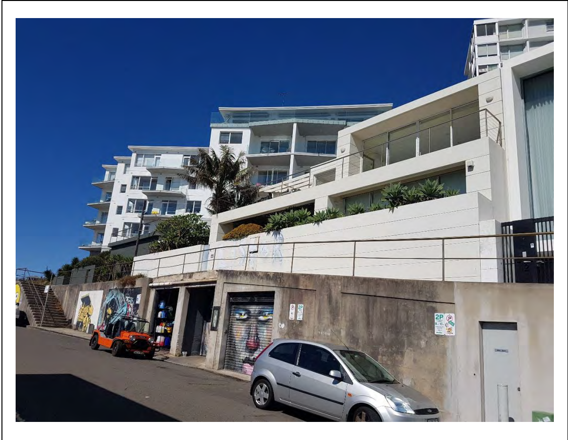
Figure 2: Site viewed from Notts Avenue
