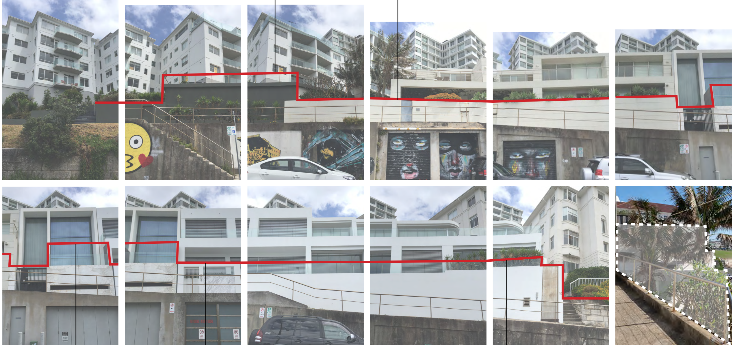
1.5 storey sheer wall and balustrade to No.16 Notts Ave's open carpark and driveway
