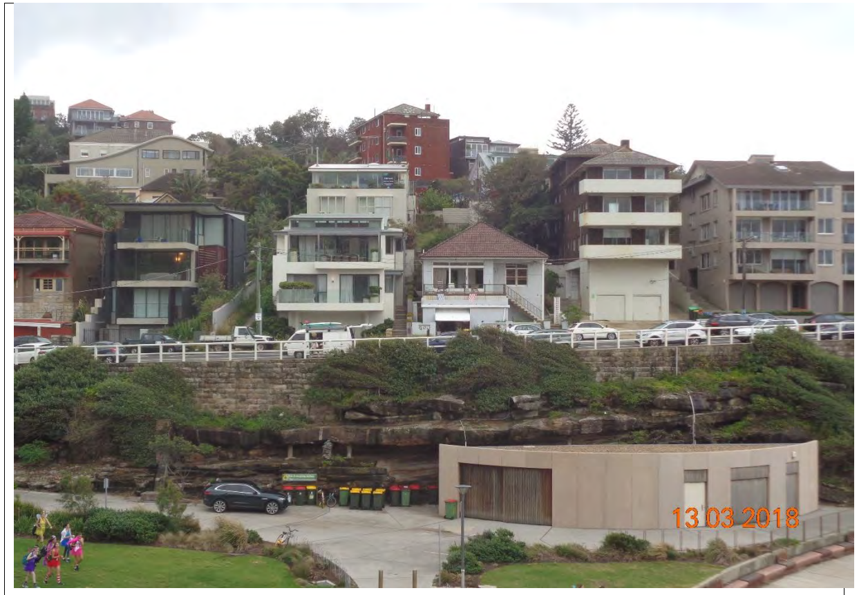
Figure 2: Site viewed from the opposite side of Tamarama Beach
