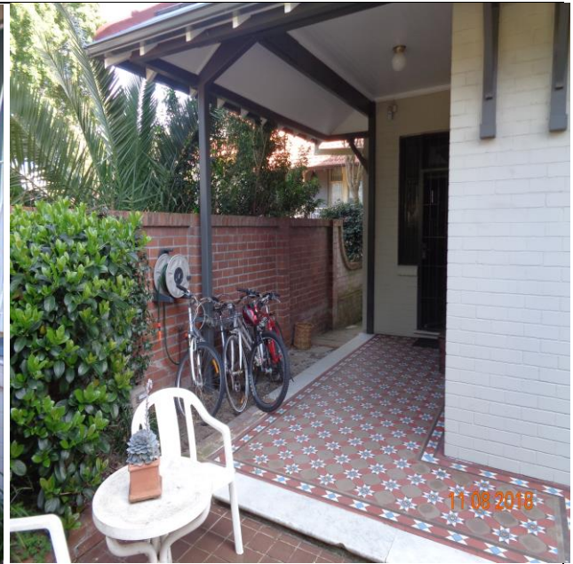
Figure 4: Front entry 2018 with dwarf wall and timber support post removed and new support post relocated to the southern side boundary.
