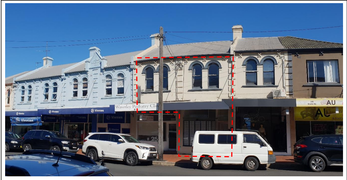
Figure 2: Subject site frontage
