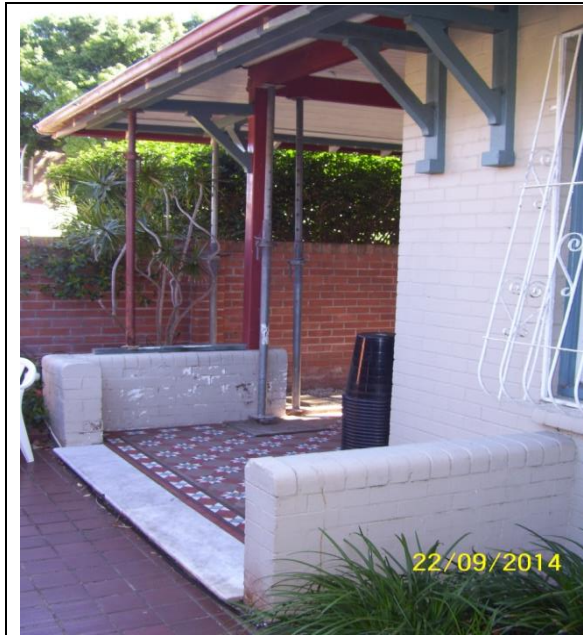
Figure 3: Front entry in 2014. Structurally unstable due to rot in structural members. Hence the temporary support posts.
