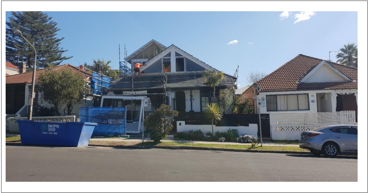
Figure 4: Adjoining properties to the left (south) – Nos 15 and 17 Barracluff Avenue
