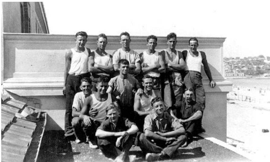
Council workers building the Bondi Pavilion, 1928.
