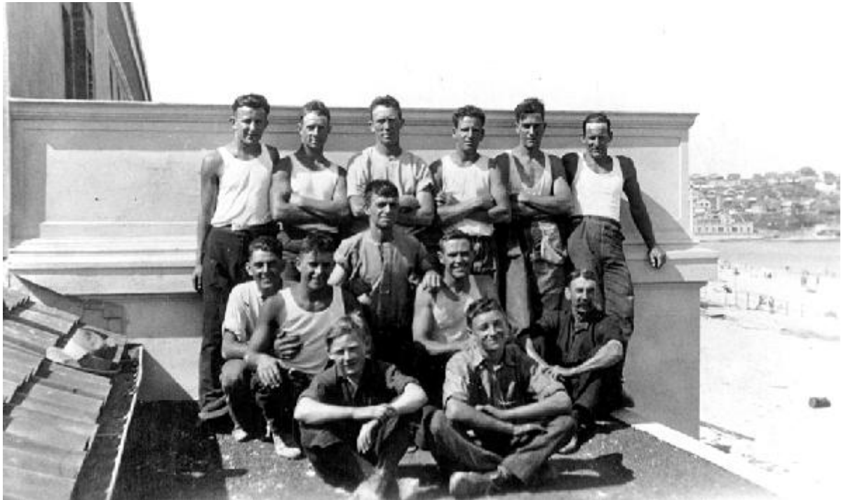
Council workers building the Bondi Pavilion, 1928.
