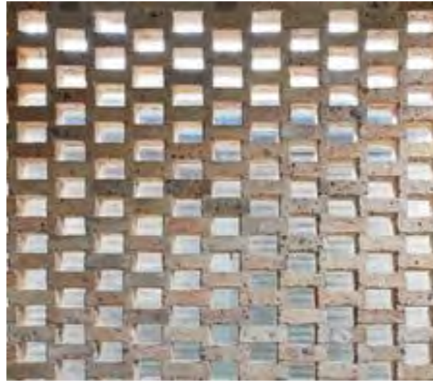
hit and miss brickwork screen
