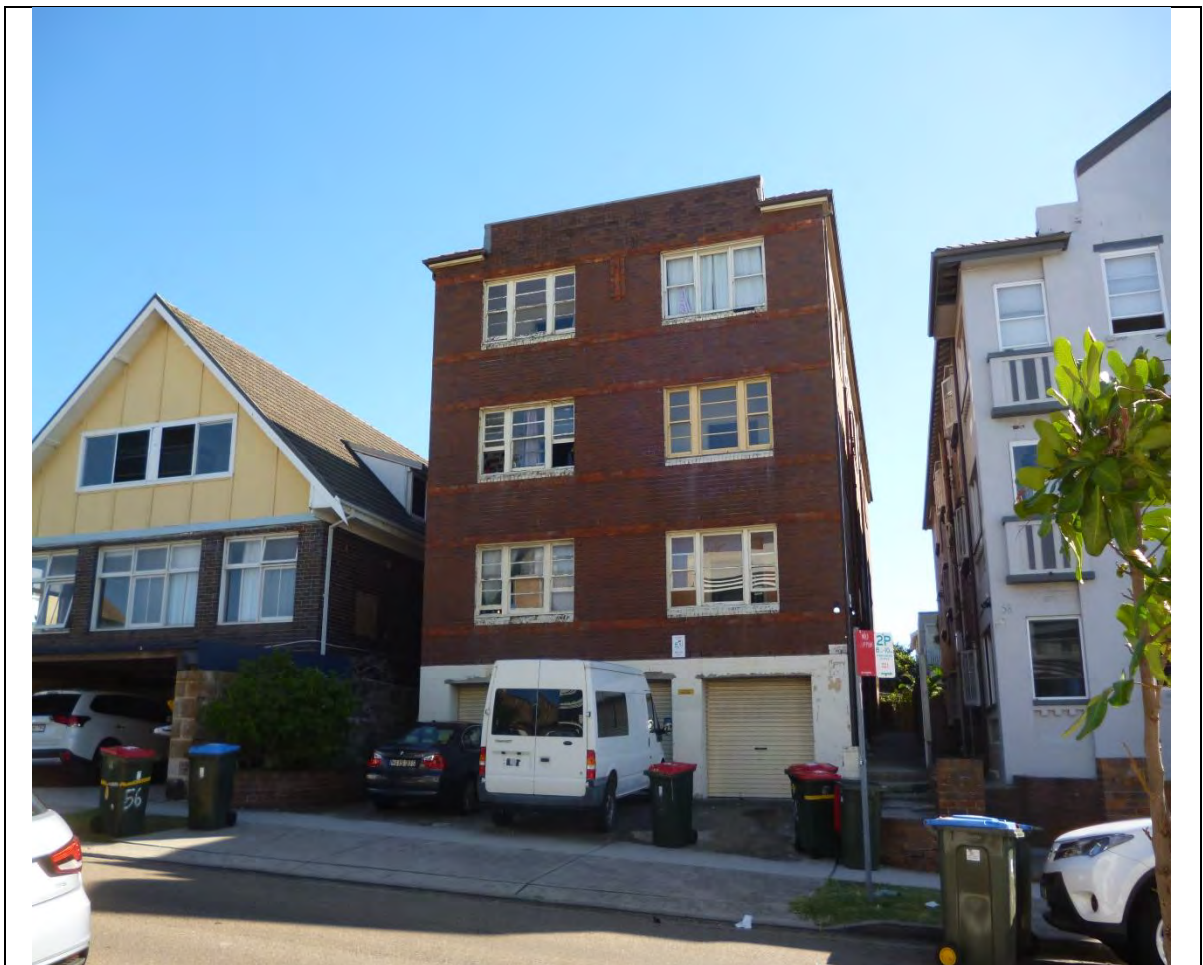
Figure 1: Subject site frontage
