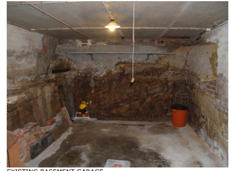
EXISTING BASEMENT GARAGE
