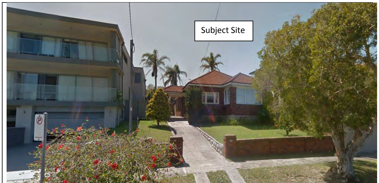
Figure 1: Site viewed from Wallangra Road
