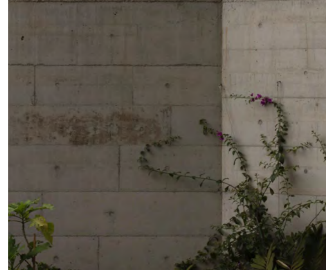
off form concrete
