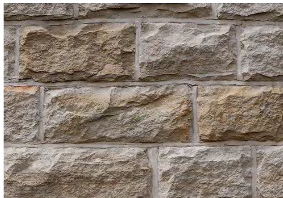
sandstone block wall to be retained
