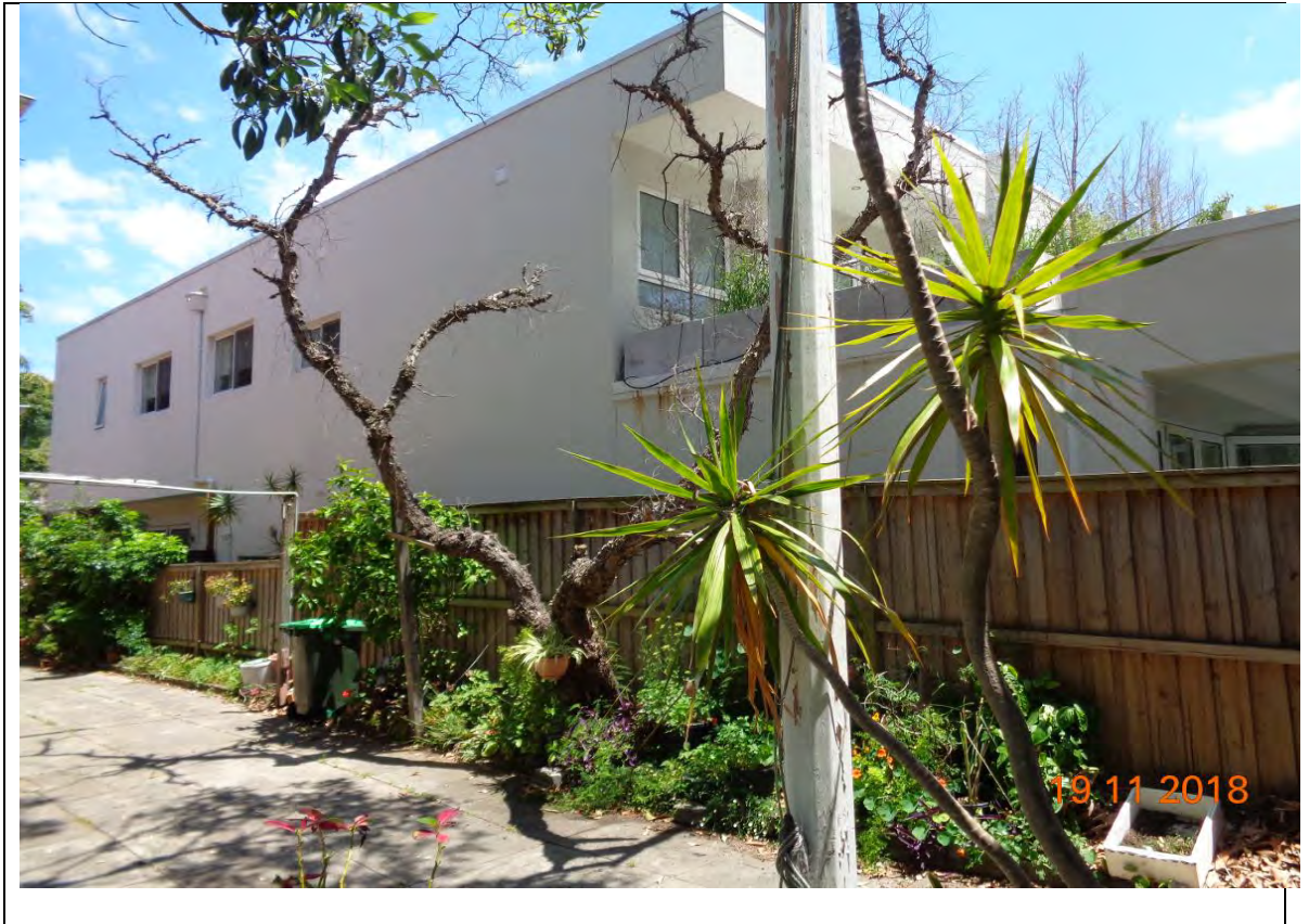
Figure 2: View of the existing dual occupancy development at 14 Owen St, to the west of the site.
